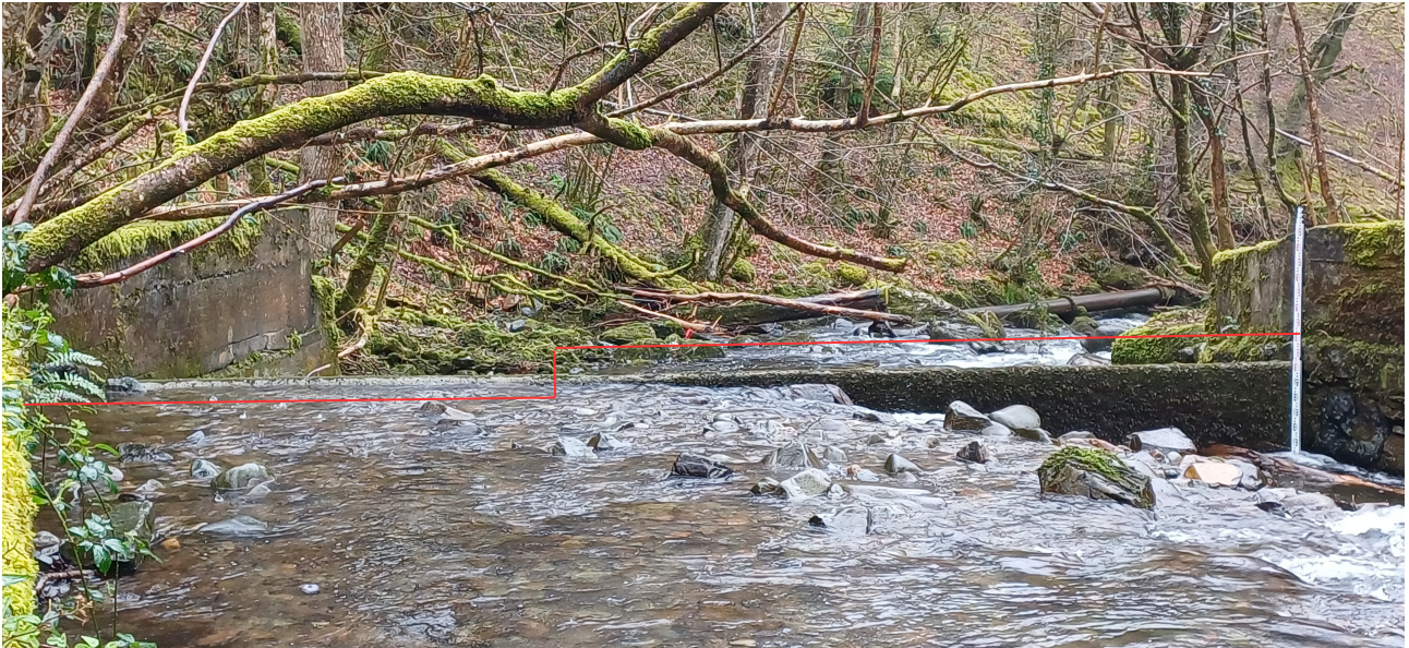
View of Main Weir Crest Looking Downstream
