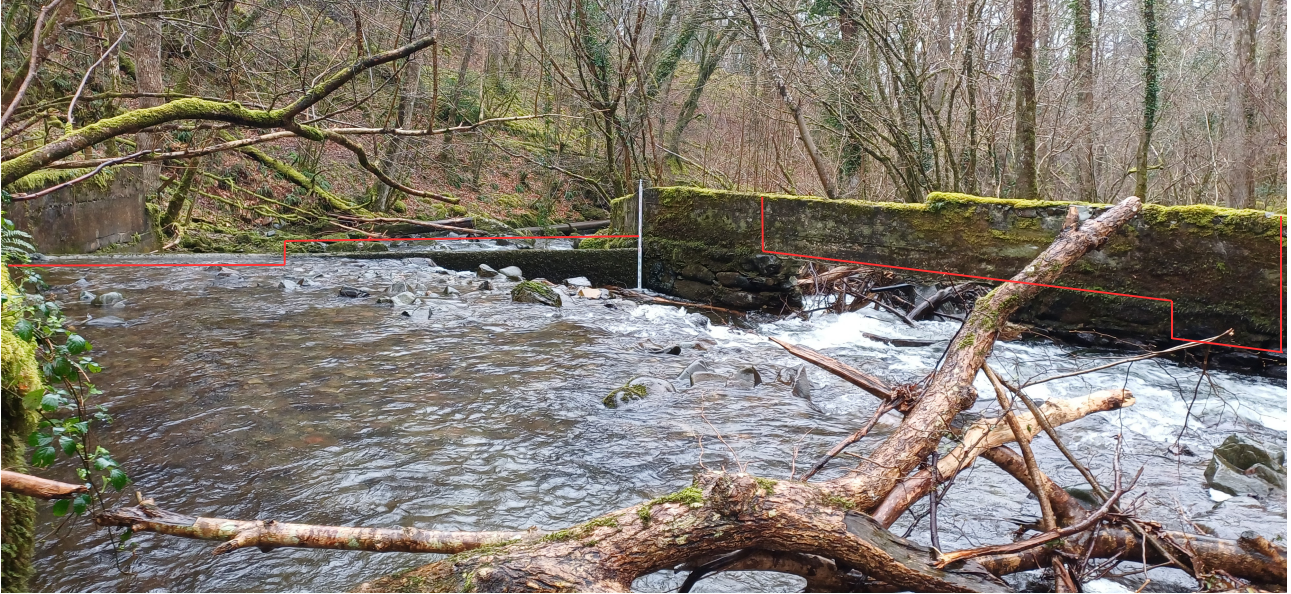
View Including Side Wingwall and Compensation Notch
