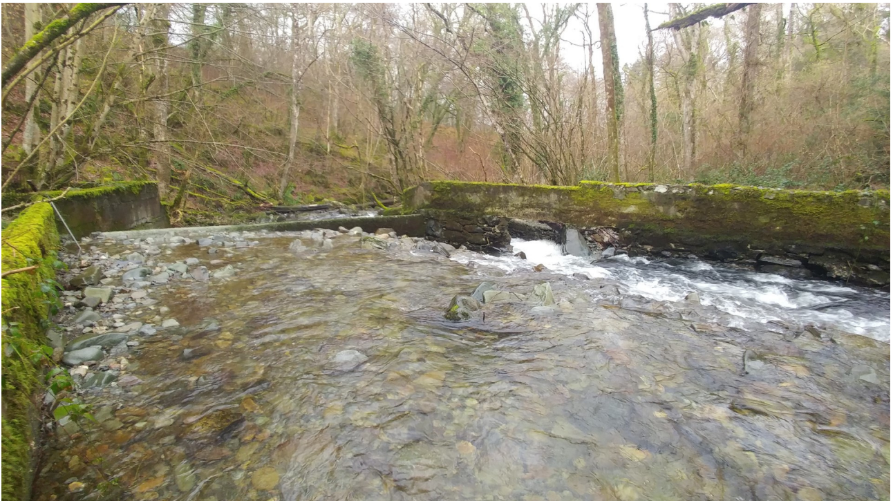
Photo 212:2 View looking downstream towards weir crest
