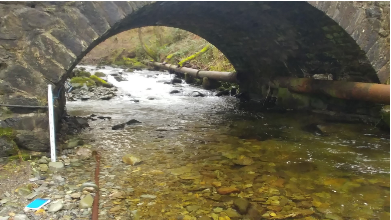
Photo 214:1 View upstream under road bridge
