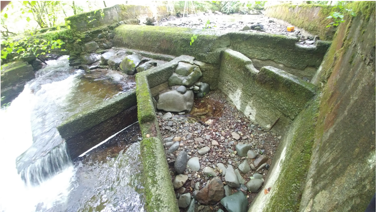
Photo 212:3 View of weir from downstream
