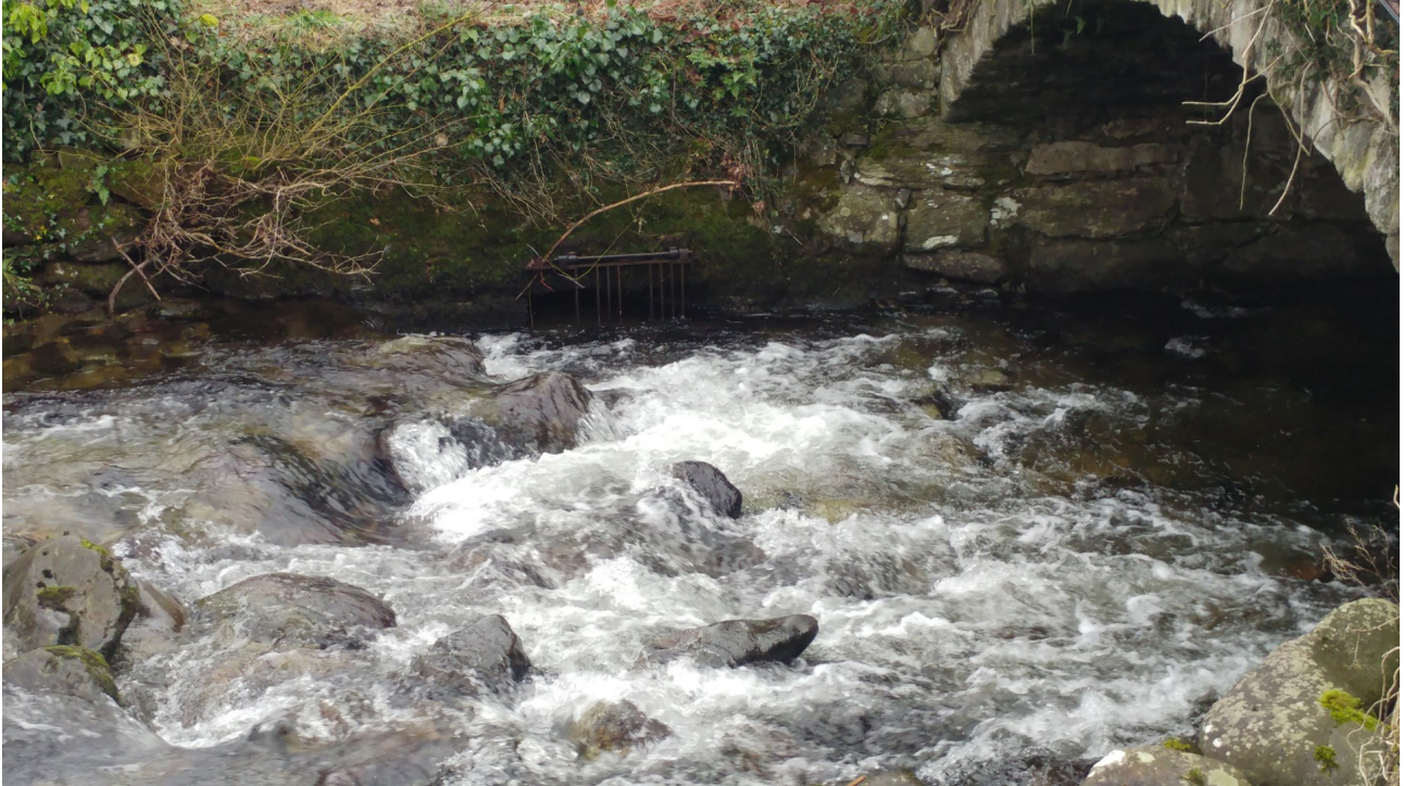
Photo 216: View West across river to existing outfall screen
