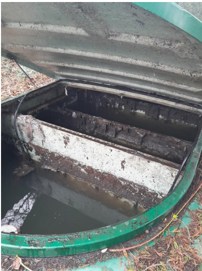
Fig 4 First chamber of the Sewage Treatment Plant
