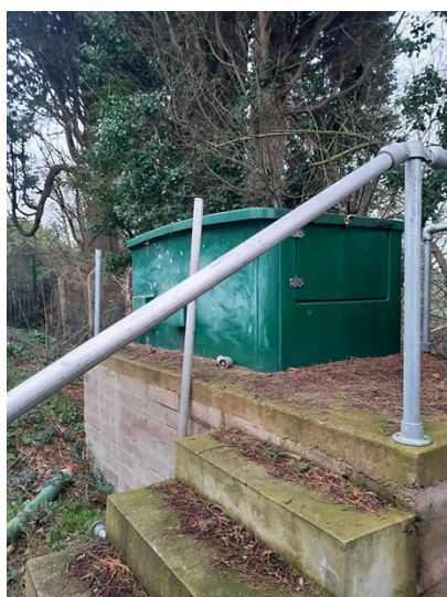
Fig 2 Sewage Treatment Plant
