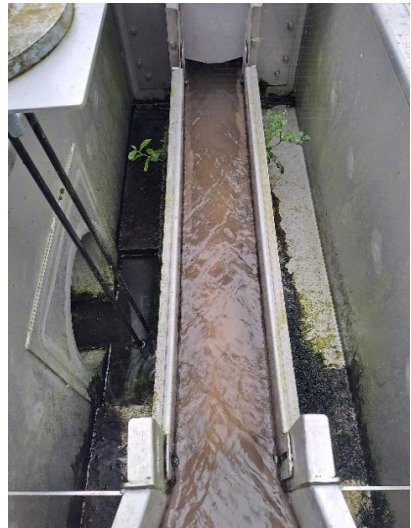
Storm Overflow Weir
