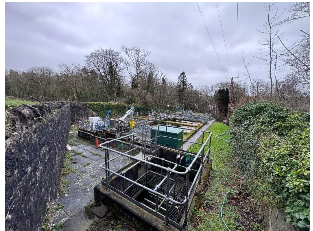
Overview of Spill Location
