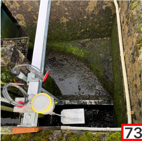
Level Sensor Location and Serial Number
