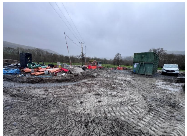
Site Under Construction ATOV
