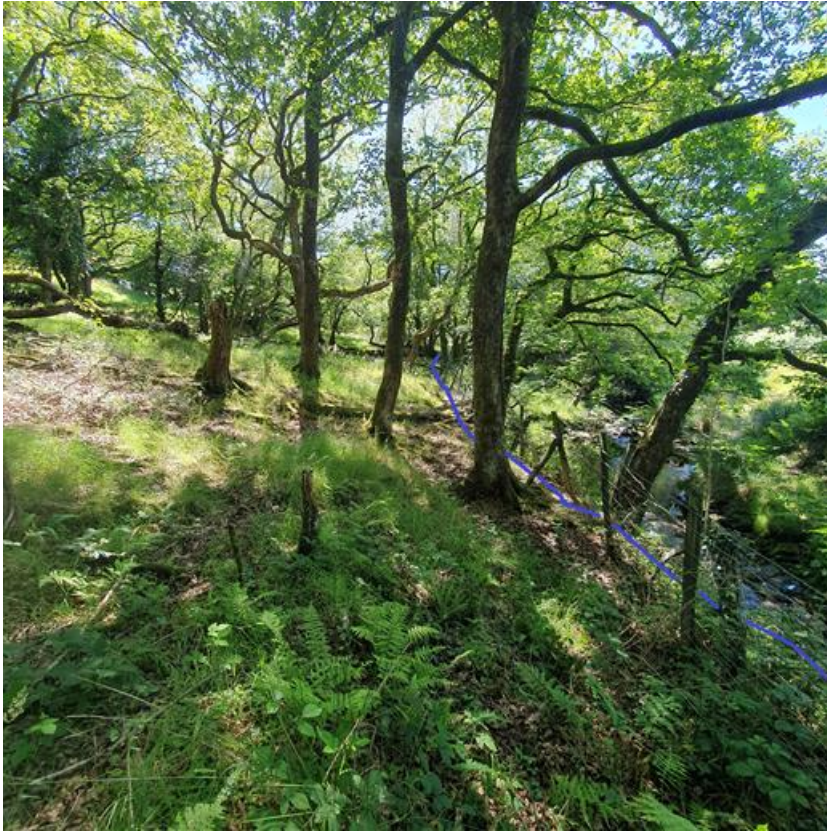
Overground pipeline at top (route shown by blue line)
