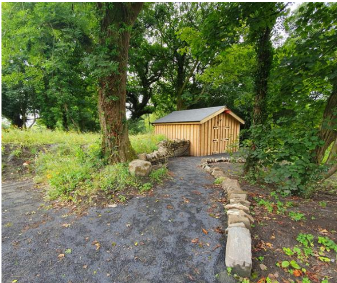
Powerhouse Location (existing)
