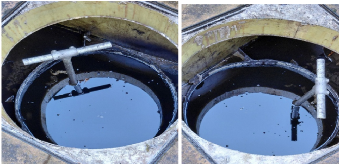
Photos 7 & 8 showing inspection chamber of the interceptor on Feb 26
