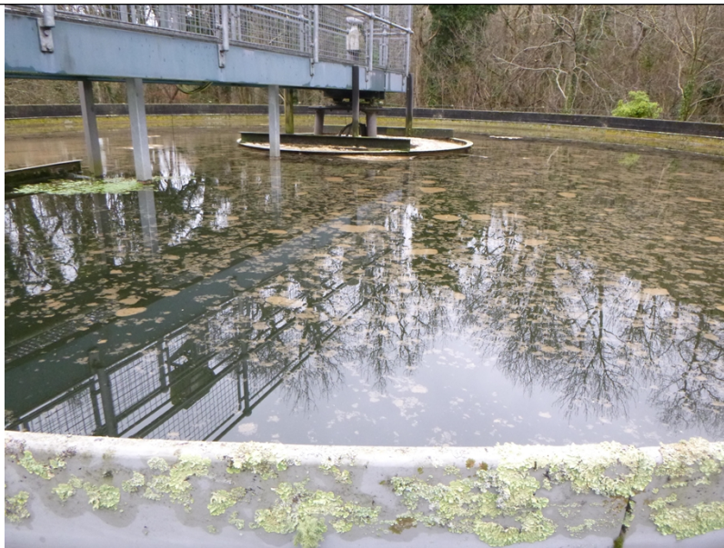
Photograph 3: One of two final settlement tanks
