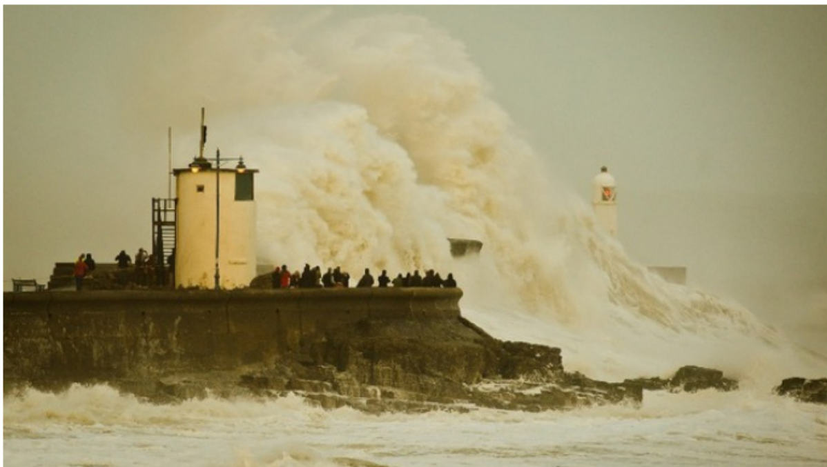
Figure 16. Wave overtopping at the Western Breakwater during a storm event on 12 February 2014
