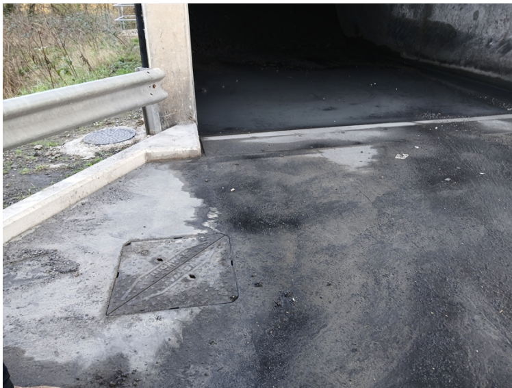
Improved kerb to prevent run-off at IBA bulk storage area
