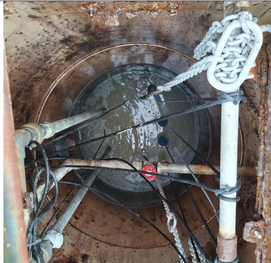
Image 2: copy of recent onsite turbidity tests
