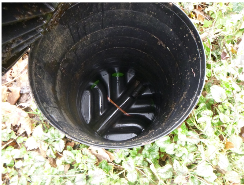
Photograph 4: Inspection chamber near soakaway
