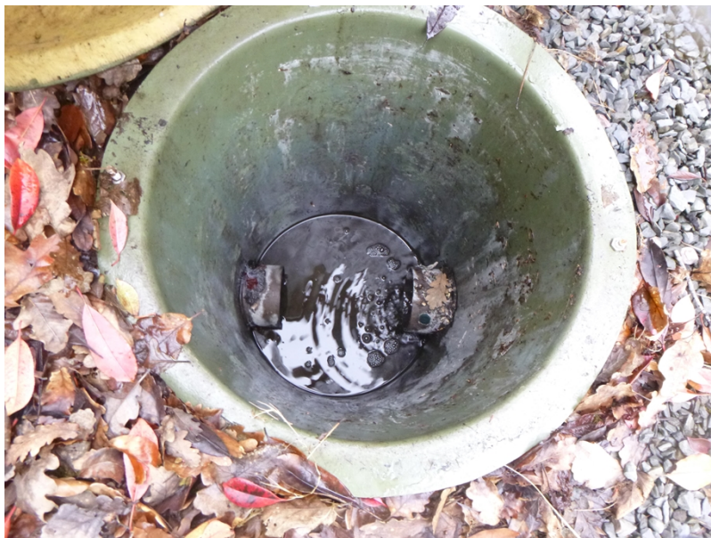
Photograph 3: Final effluent sample point
