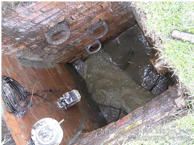
Image 1: CSO chamber with flow overtopping overflow structure
