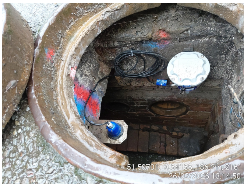
Image 1: Overflow pipe within chamber
