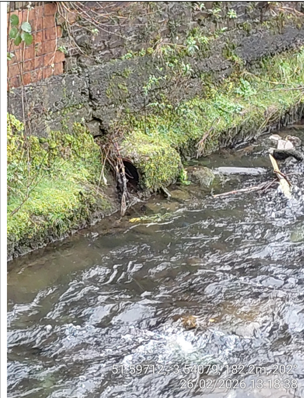
Image 2: Outfall pipe to the watercourse
