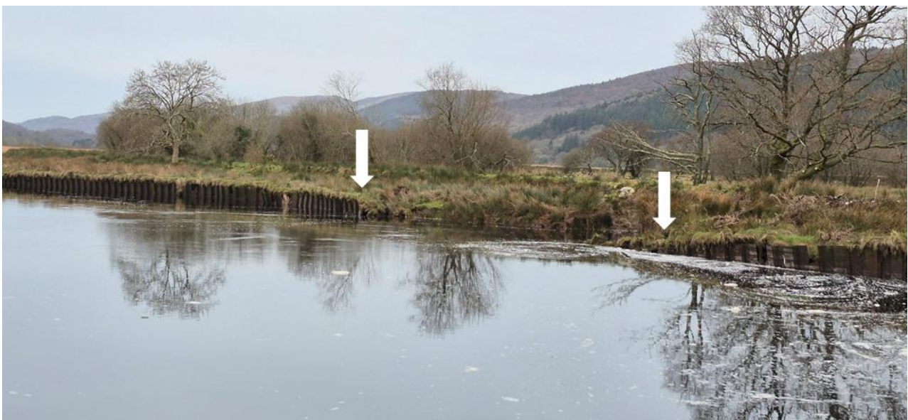
Figure 3-3 Shows the section of failed sheet piling (between white arrows) on the Afon Mawddach (right bank looking downstream, SH 71235 19076)
