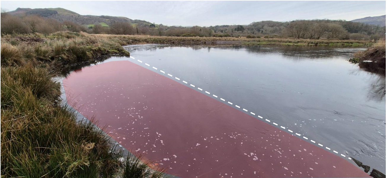
Figure 3-4 Shows the section of failed sheet piling and the extent of subsequent lateral channel movement and scour. White line represents where the existing bank line and sheet piling was. With the red area representing the extent of scour (right bank looking upstream, SH 71174 19069).
