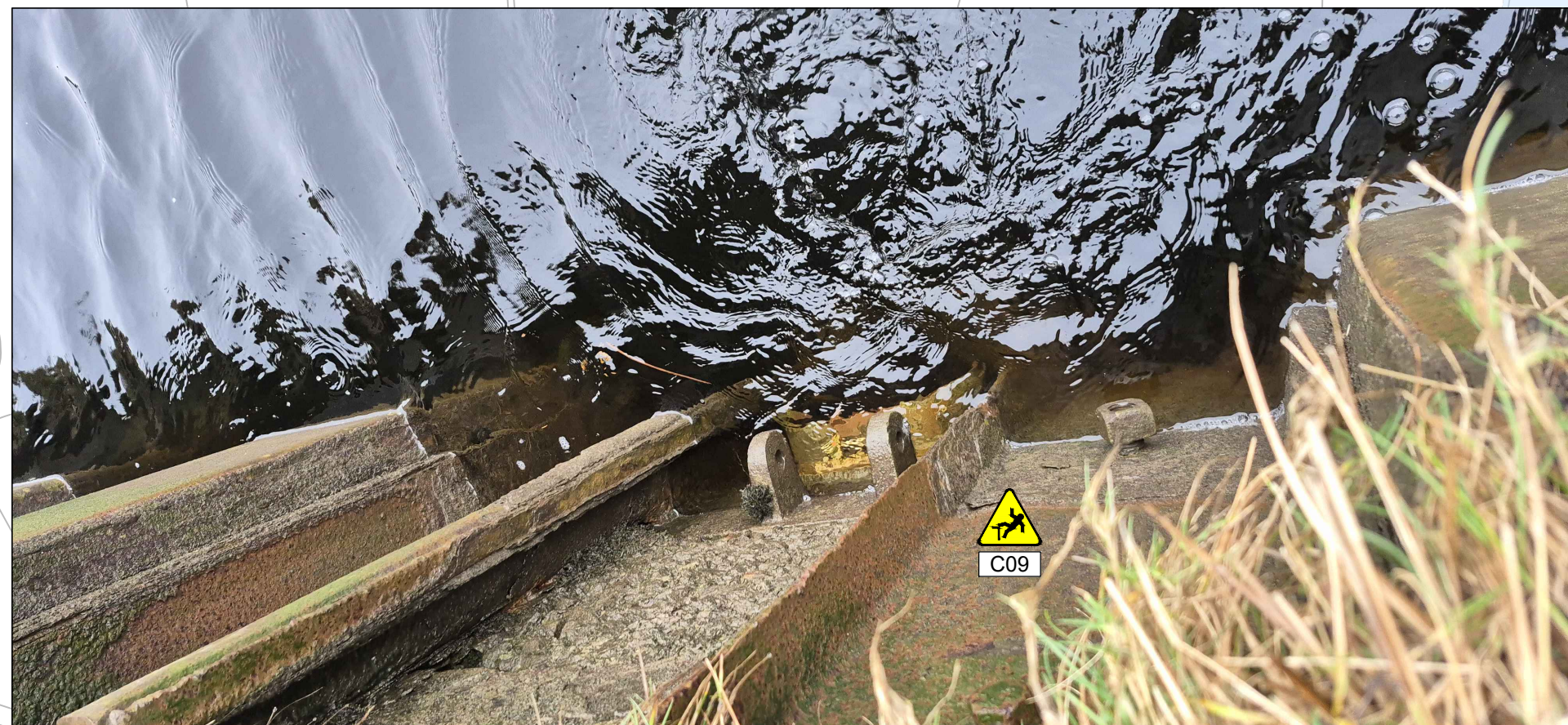
FIGURE 3 EXISTING OUTFALL IN SHEET PILE WALL
