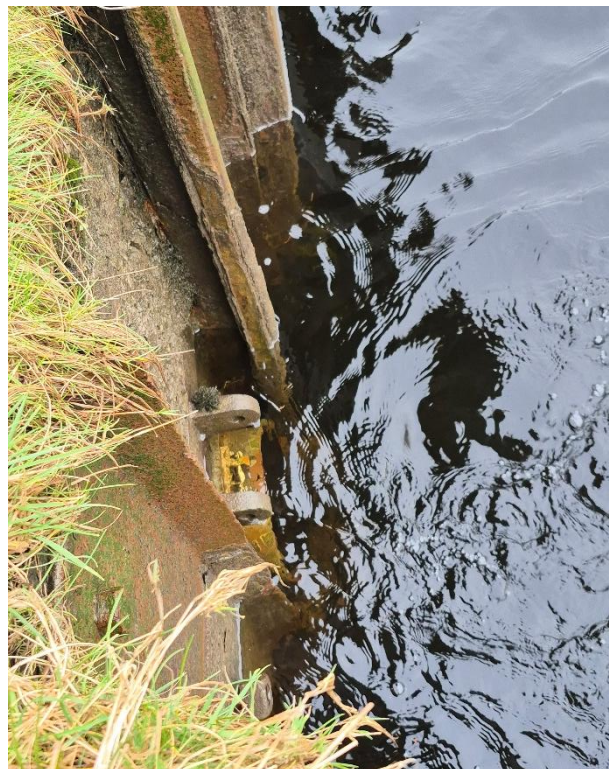
Figure 3-6 Outfall in the sheet piling missing a flap valve (right bank looking upstream).
