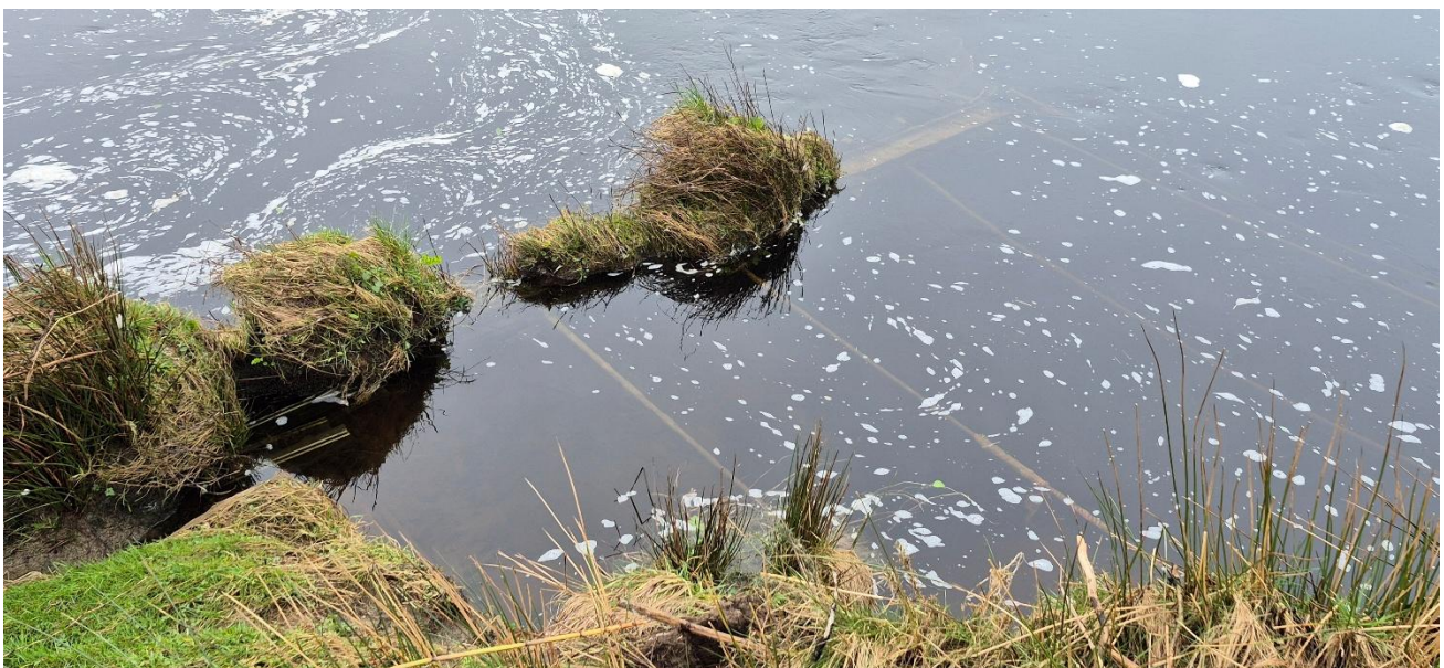
Figure 3-4 Foundation tie rods of the failed sheet piles still in place, just visible below the high tide (right bank looking downstream)
