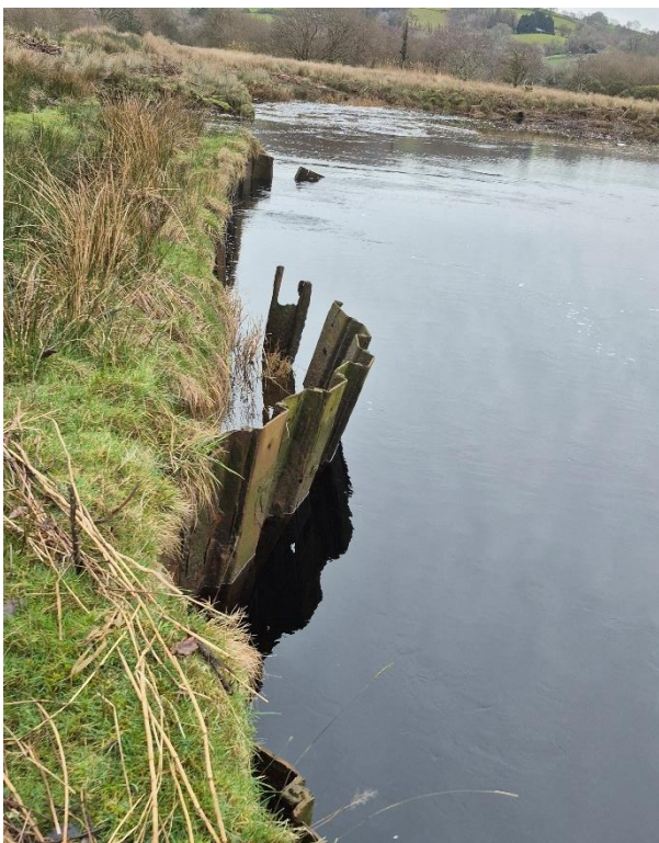
Figure 3-5 The downstream section of sheet piling beginning to fail (right bank looking upstream).
