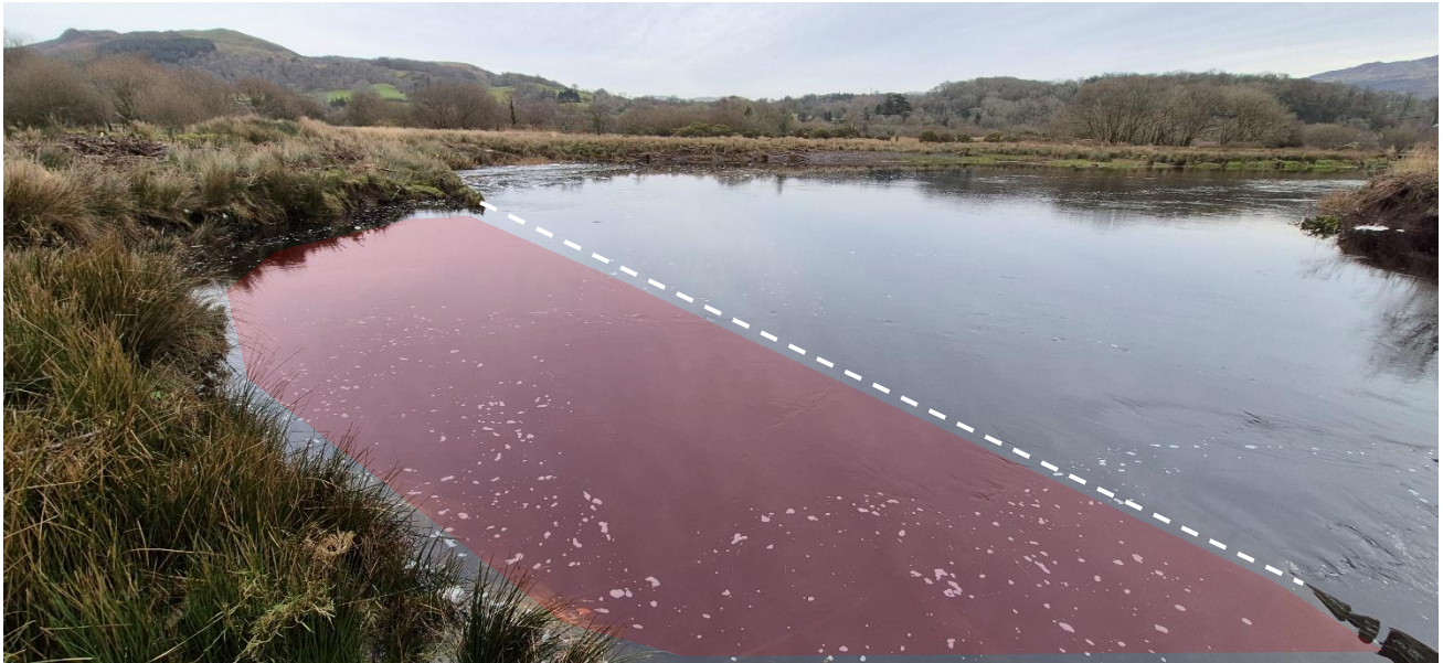
Figure 3-3 Section of failed sheet piling and the extent of subsequent lateral channel movement and scour. White line represents where the existing bank line and sheet piling was, with the red area representing the extent of scour. (right bank looking upstream)
