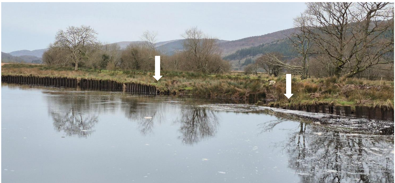
Figure 3-1 Section failed sheet piling in the middle of the image between the white arrows (Left bank looking downstream)
