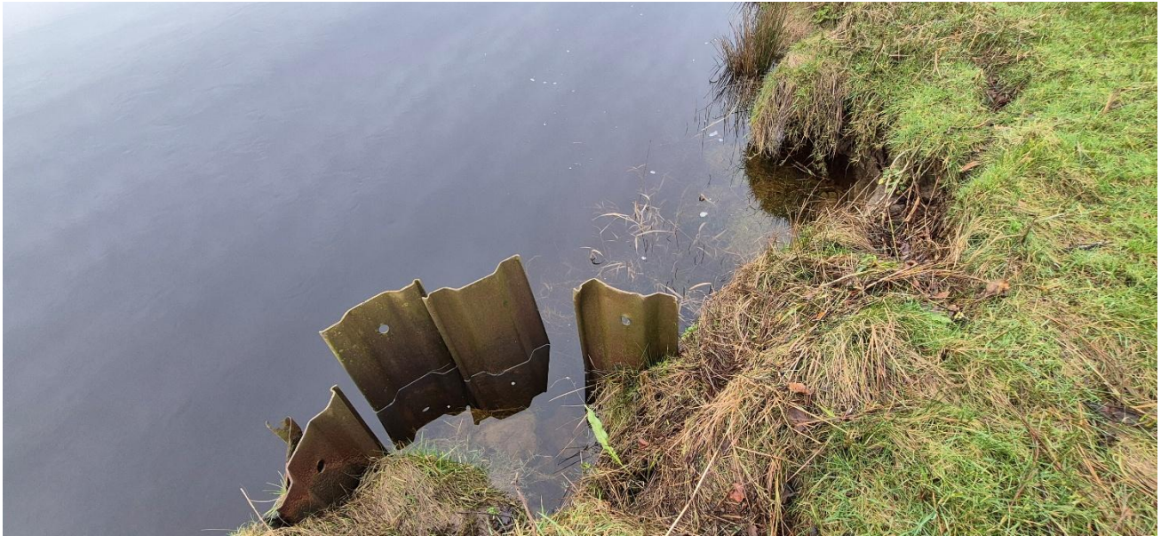
Figure 3-11 Evidence of basal scour and slumping causing deterioration and failure of the sheet piling at the downstream end of the site (right bank looking downstream)
