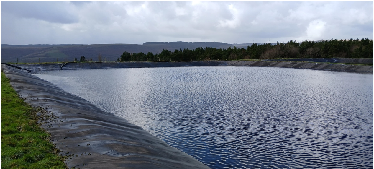
Photo 4 - Leachate pools at Bryn Pica Landfill
