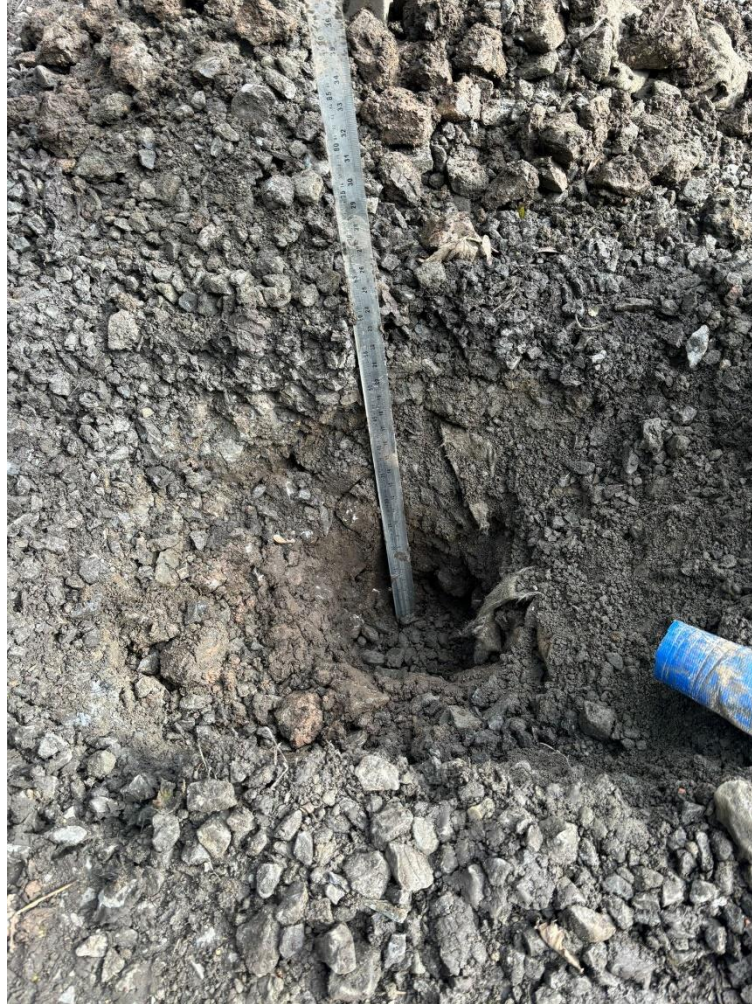
Figure 2 - Test pit F1 during excavation
