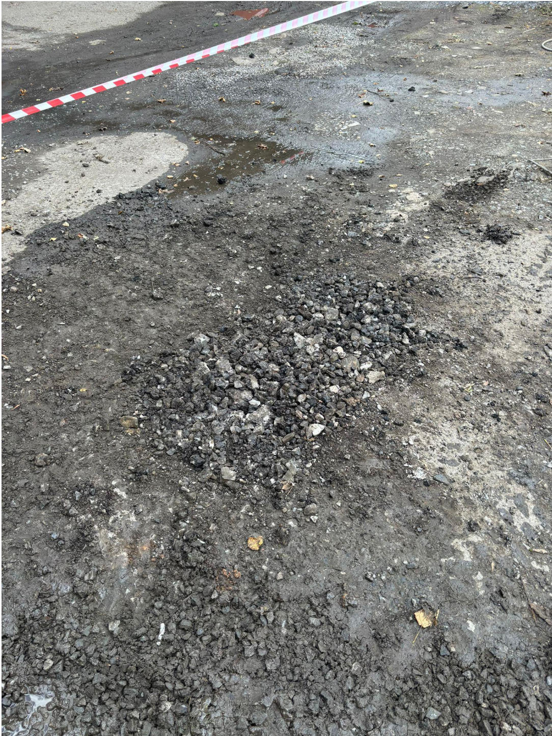
Figure 6 - Test pit remediation
