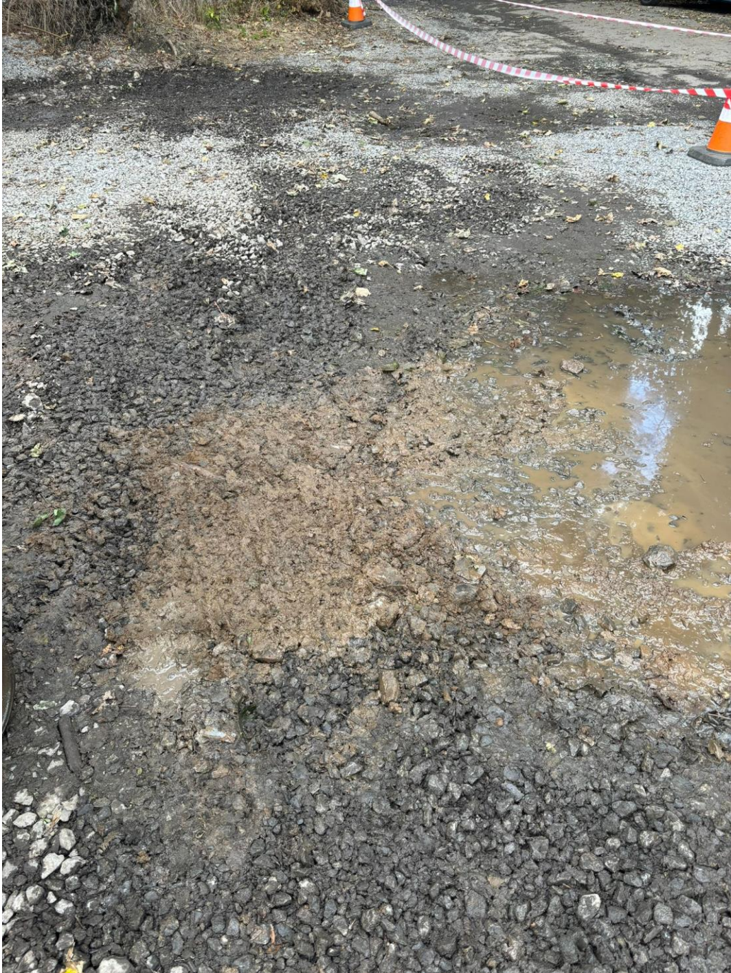
Figure 5 - Test pit remediation
