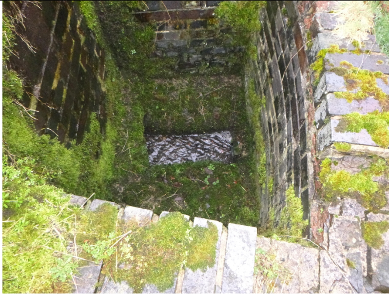
Photograph 3: Outflow from filter bed
