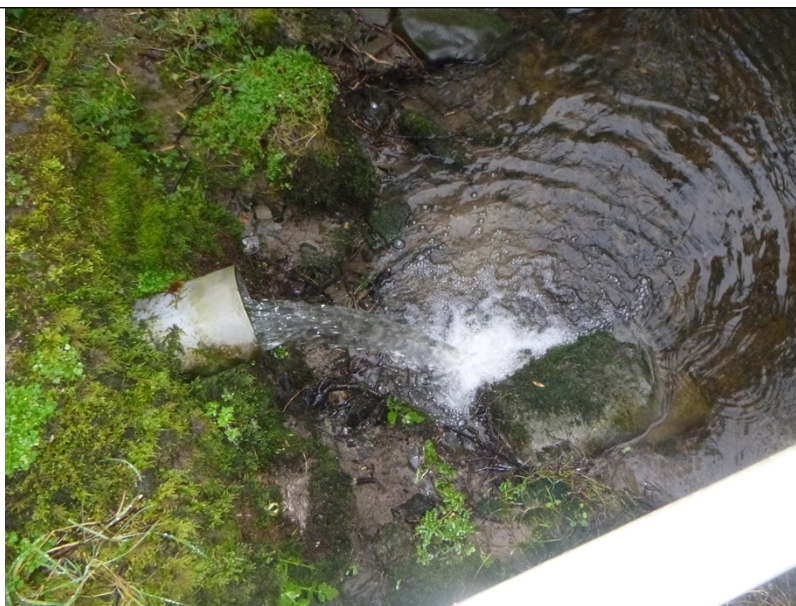
Photograph 5: Final effluent discharge point into the Afon Arth
