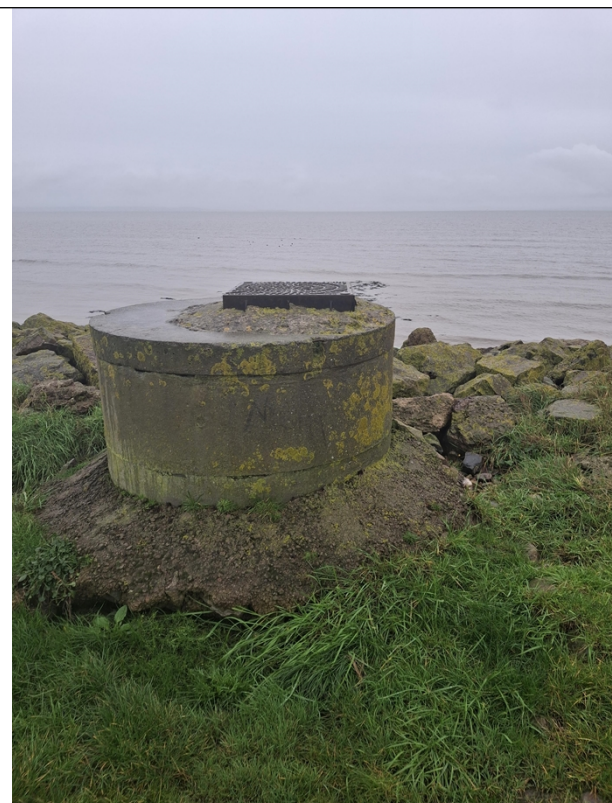
Figure 4: Point of inspection near discharge point
