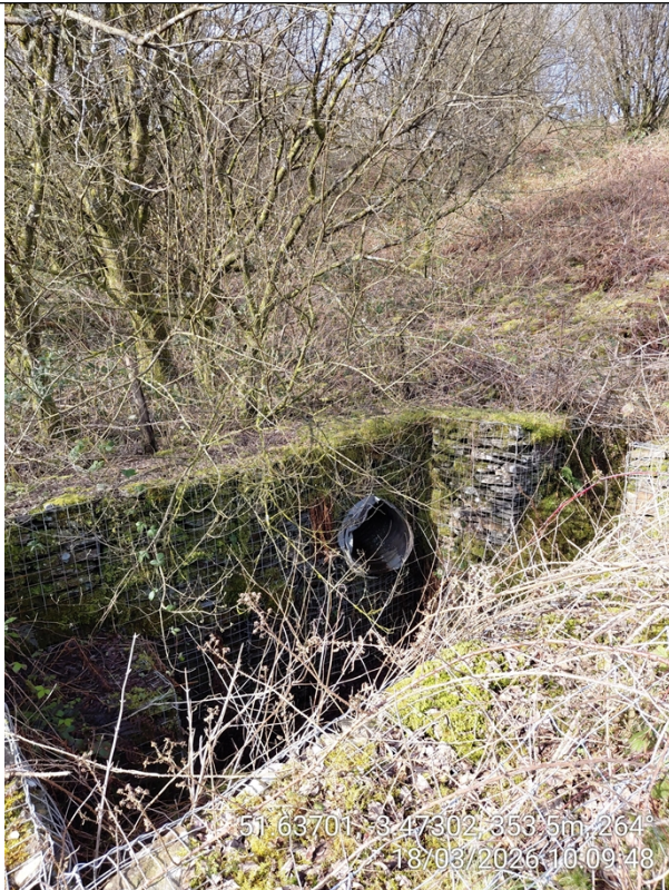
Image 2: overflow from settlement lagoons
