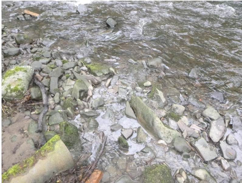
Photograph 3: Storm discharge point into the Afon Arth at SN 50867 63020
