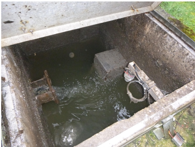
Photograph 2: Chamber following the septic tank
