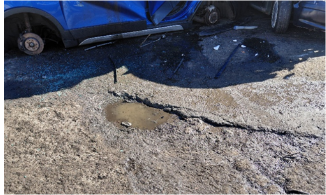
Photo 3 & 4. Area of impermeable surface showing signs of wear
