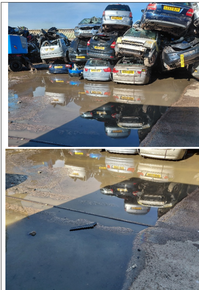
Photo 1 & 2. Photo of area where impermeable surface is allowing pooling water
