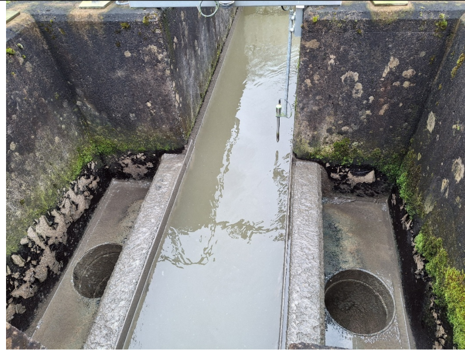
Image 01: Inlet channel showing flow not overtopping to storm tanks.
