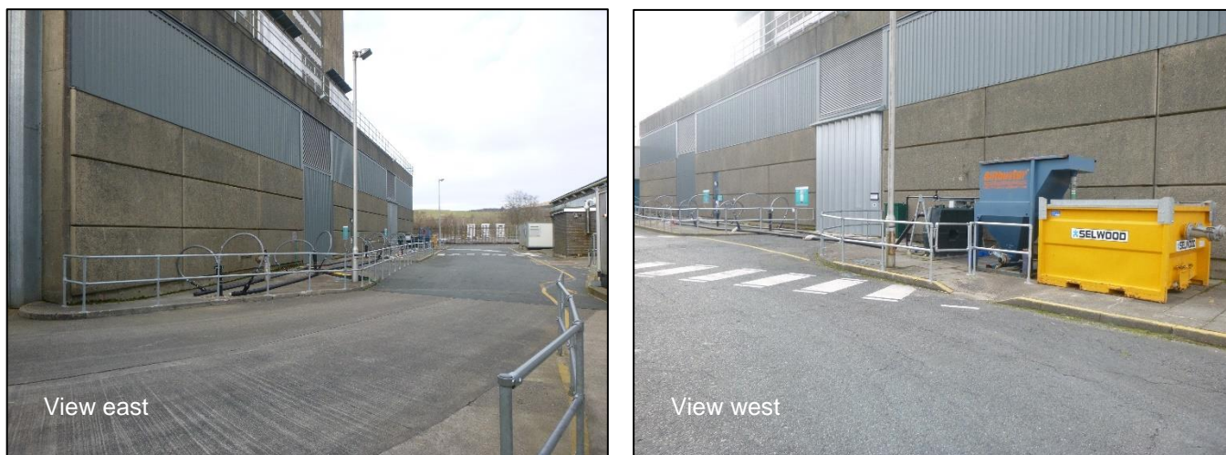
Figure 3: Photographs of the Dewatering Boreholes and Water Tanks
