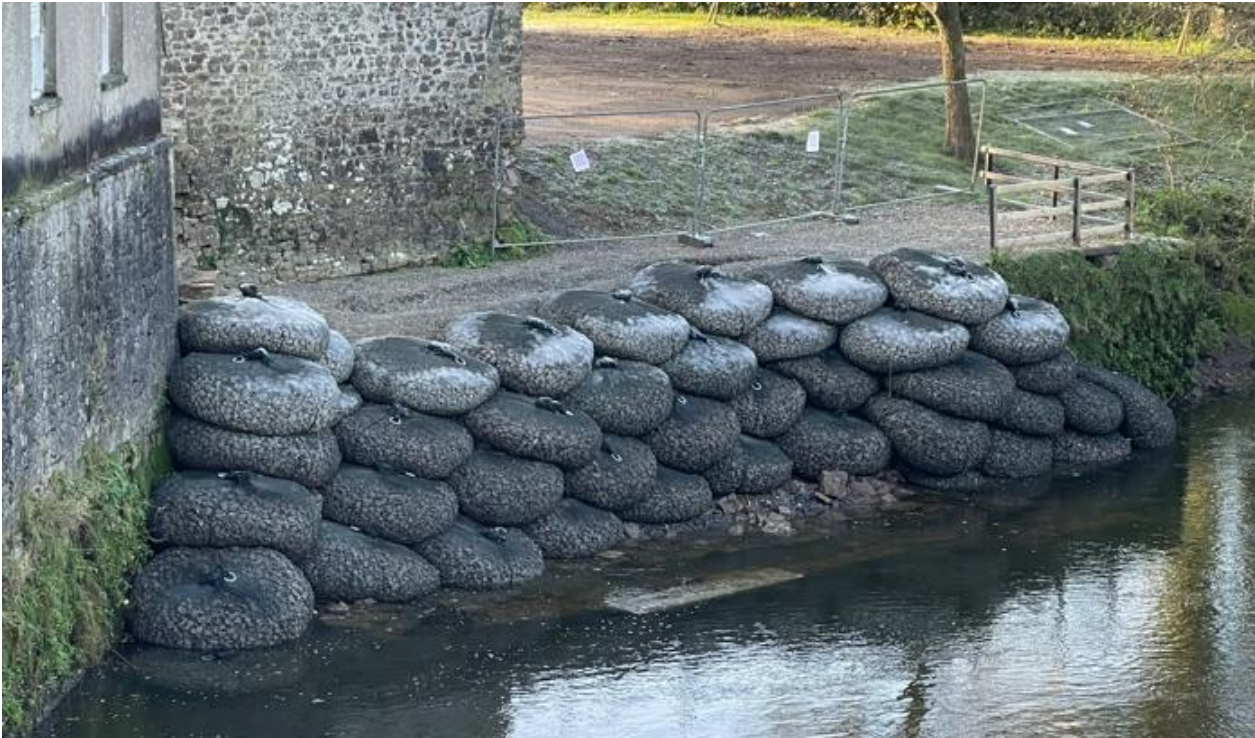
Figure 1-2: Emergency repair works to wall failure
