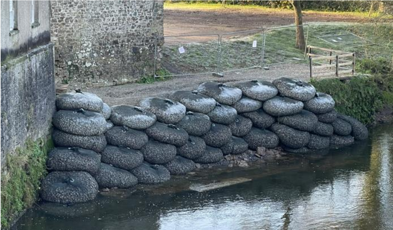
Figure 3-2: Emergency repair works to wall failure
