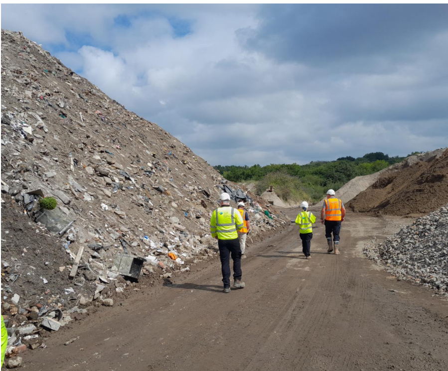
Photographs above shows construction and demolition waste which is being used to produce the
