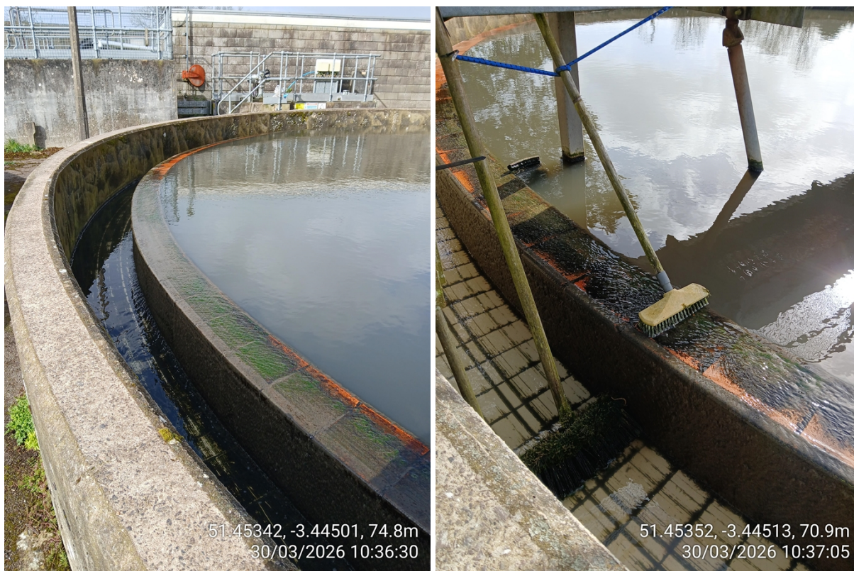
Left: FST 2 with some fungus build up on the tiles. Right: FST 2 ineffective brushes in action.
