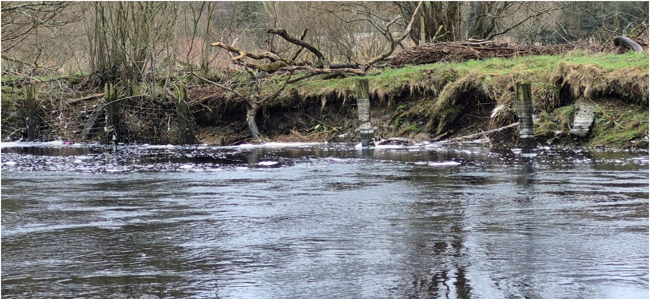
Figure 3-10 Section of eroded bank face between the Afon Mawddach and the Afon Wnion. A fence/ failed bank protection is visible in the form of posts in front of the bank face
