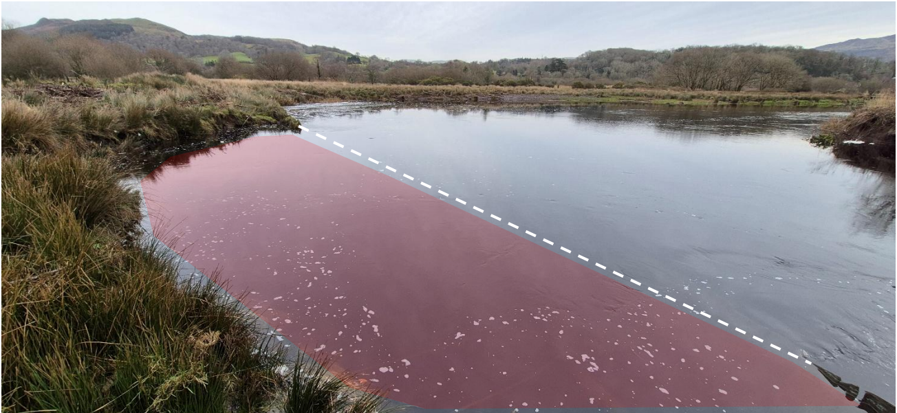
Figure 3-3 Section of failed sheet piling and the extent of subsequent lateral channel movement and scour. White line represents where the existing bank line and sheet piling was, with the red area representing the extent of scour. (right bank looking upstream)
