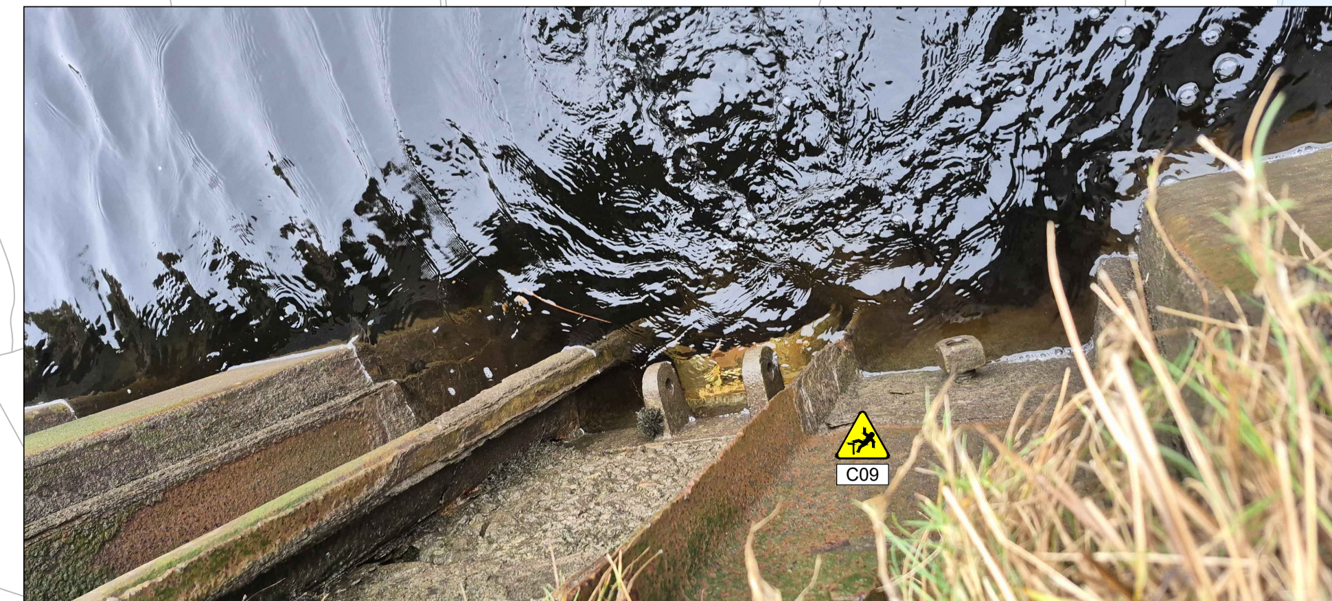
FIGURE 3 EXISTING OUTFALL IN SHEET PILE WALL
