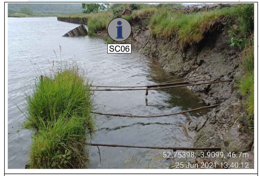
FIGURE 2 EXPOSED GROUND ANCHORS
