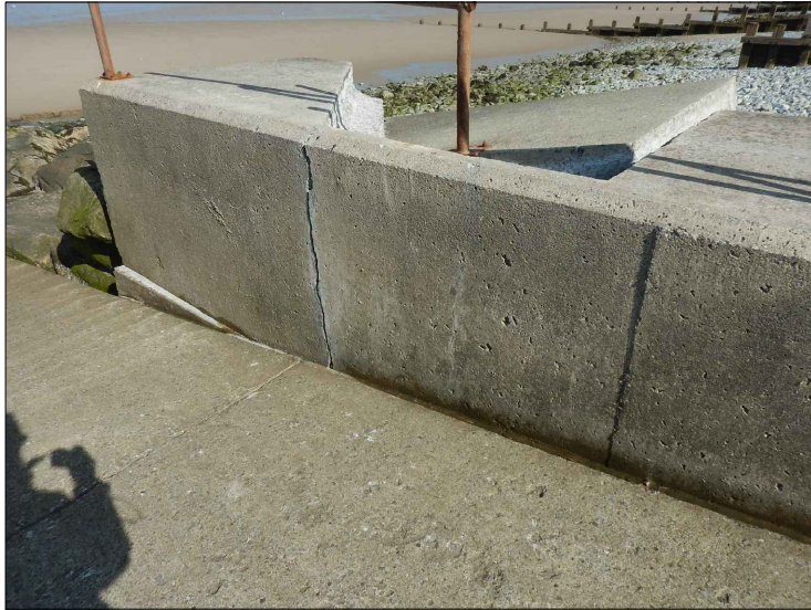
Back of Outfall
