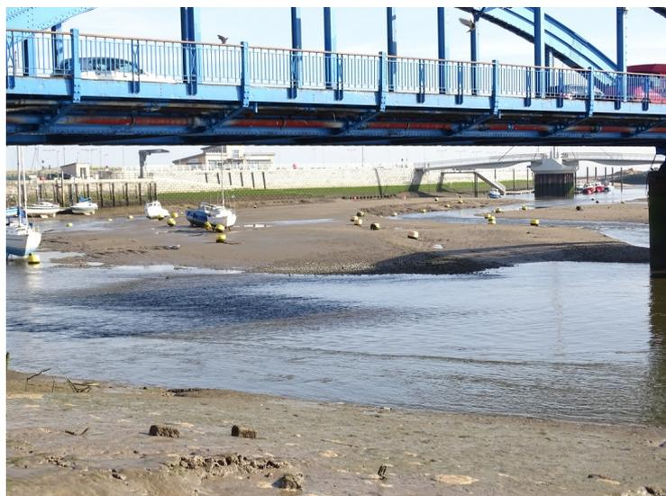
**Area 2** – Area under the footbridge and central pontoon – this has an average volume of 3,081m<sup>3</sup>. This area requires a level of -1.5mAOD to allow access to the main navigation channel and pontoon areas.
