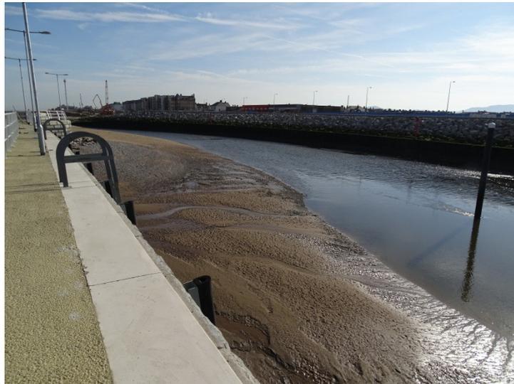
The material to be dredged is predominantly building up around the turning circle which accounts for approximately 6000m<sup>3</sup> of material to be removed. The previous modelling indicated that the material was likely to build up in this area however not to the extent that has been observed recently. This is explained further In our response to question 2.
