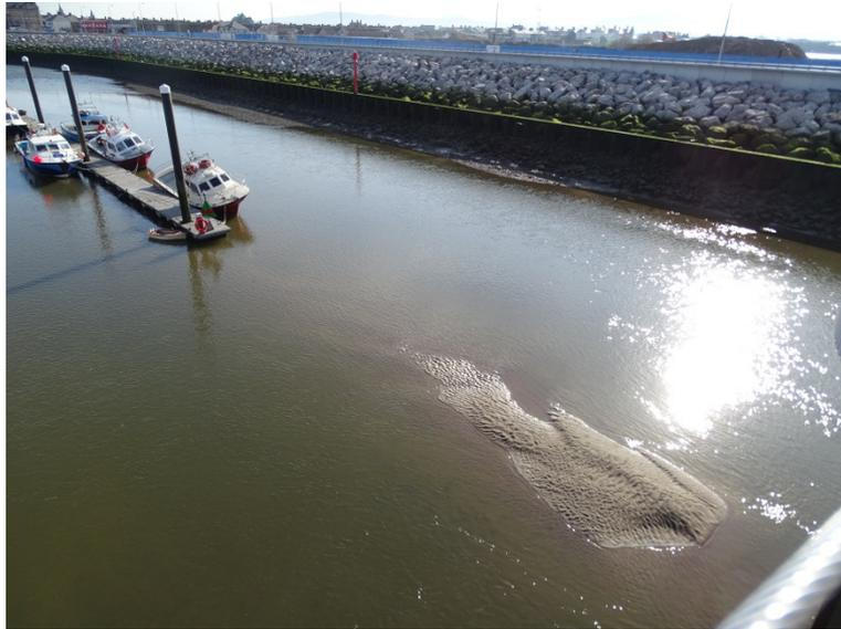
**Area 3** – the turning circle – this has an average volume of sand to be removed of 6,000m<sup>3</sup>. This volume of material is required to be removed to allow access to the navigation channel and the fenders on the quay wall. Without this removal of sand the harbour is not fulfilling its requirements.
