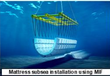
Mattress subsea installation using MIF
