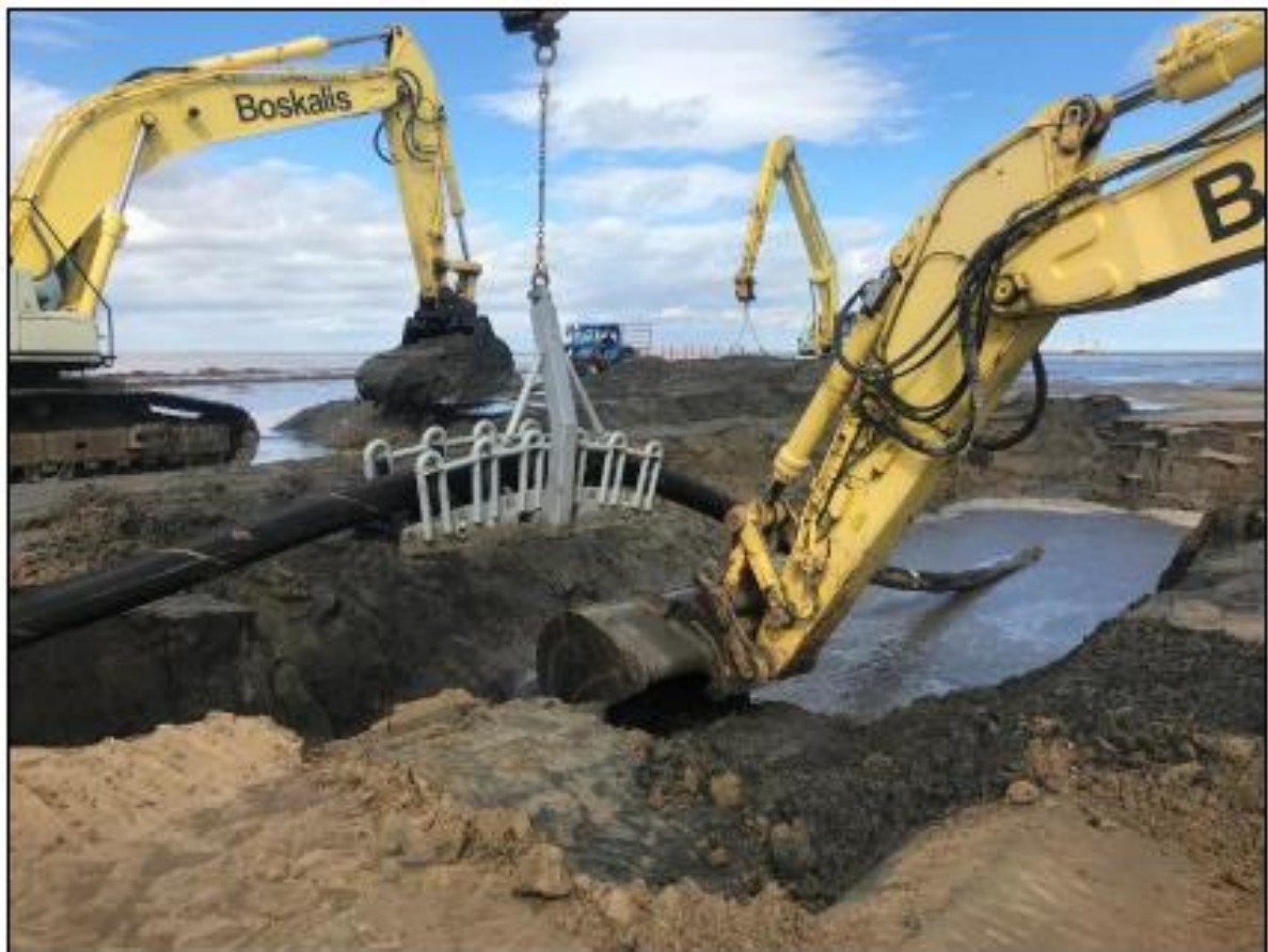
Figure 2.11: Digging from both sides of the cable
