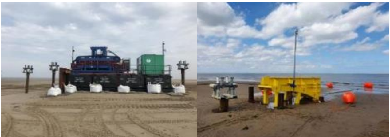
Figure 2.6: Cable tensioner pontoon (left), and shoreline beach chute (right)
