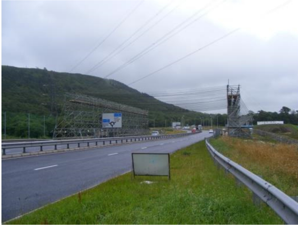
Figure 2.4: A Netted Scaffold Protecting A Road
