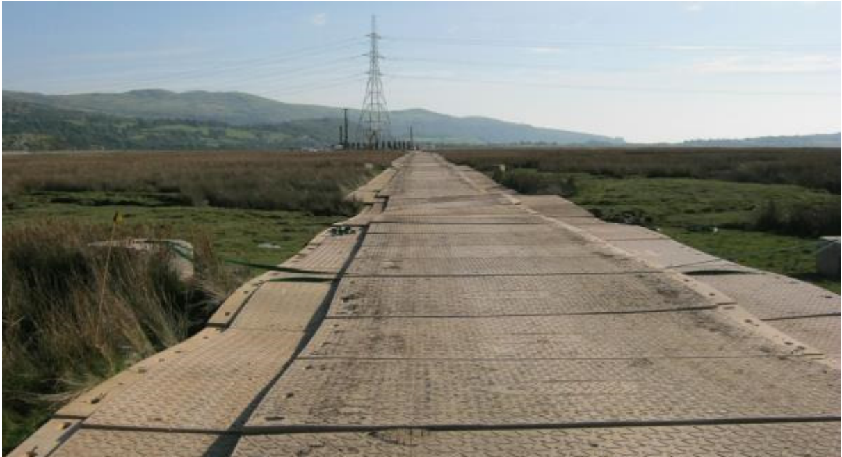
Figure 2.9: Temporary Roadways Using Plastic or Metal Panels
