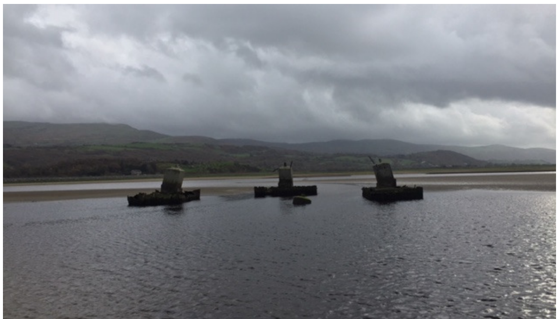
Figure 2.7: Redundant 4ZC030 Foundations at Low Tide Showing Chimney and the Top of the Pile Cap
