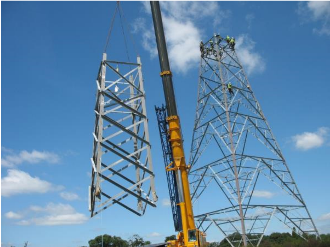
Figure 2.3: Pylon Erection at Upper Levels
