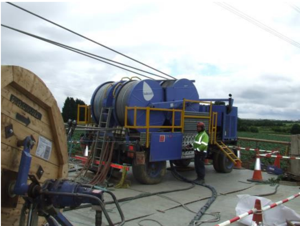
Figure 2.10: Operational EPZ Constructed from Aluminium Panels
