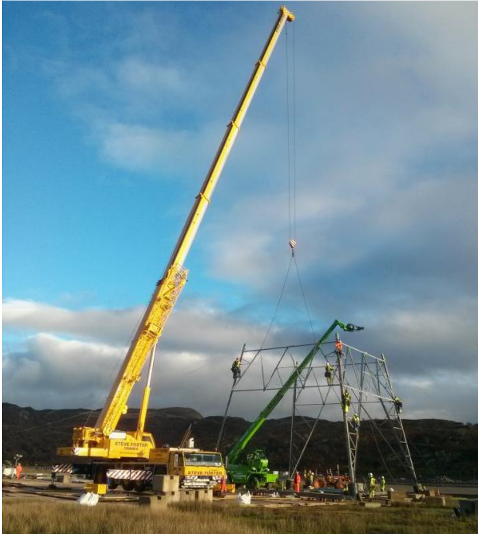
Figure 2.2: Pylon Erection at Base Level
