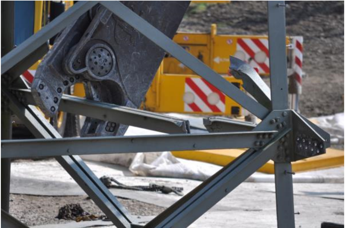
Figure 2.5: Hydraulic Shearer Mounted on an Excavator Boom
