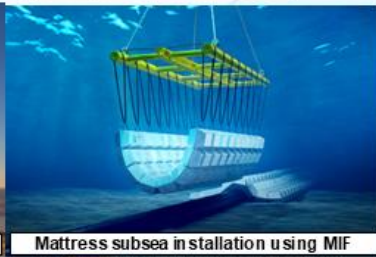
Mattress subsea installation using MIF
