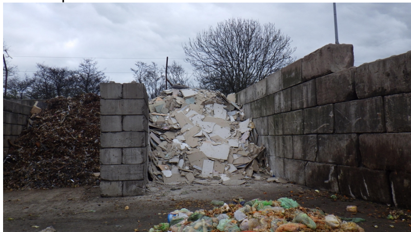
Plasterboard stored in open bay ACTION: Plasterboard to be removed from this bay and stored in a sealed, weatherproof container by Friday 22nd May 2026
