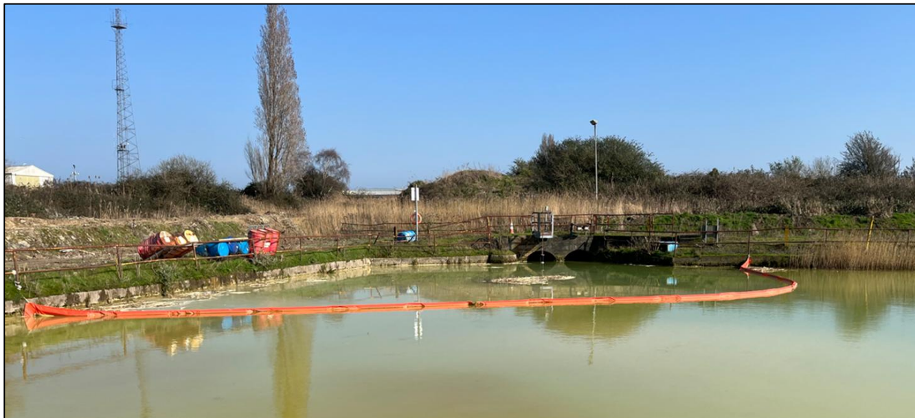
Photograph 3. Lagoon 14 and revised oil/hydrocarbon control boom arrangement,
