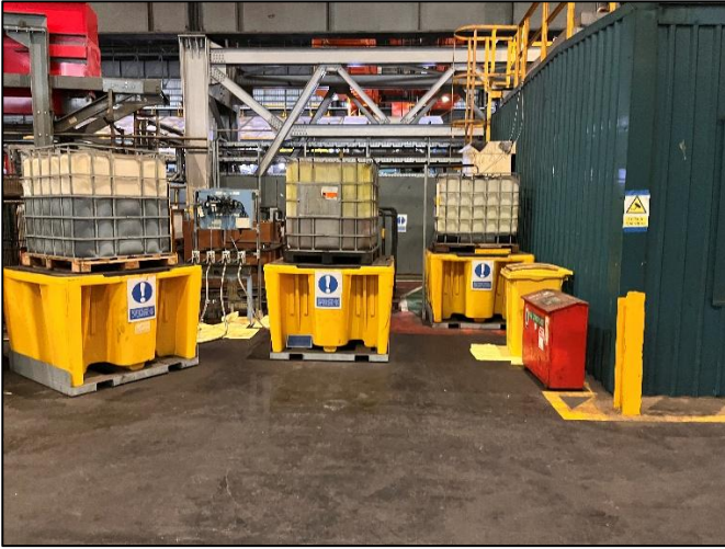
Photographs 1 & 2. Oil storage arrangements at the Automotive Finishing Line (AFL)
