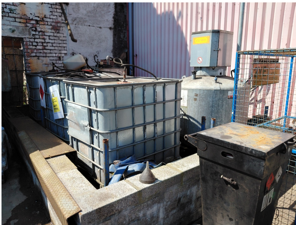
Image 3: Segregated ELV fluids in labelled containers.
