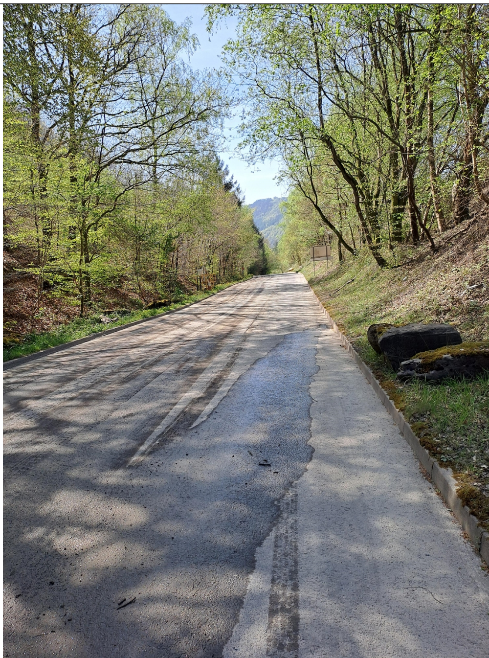
Figure 3 – Runoff observed leaving site and entering a road drain during the visit.
