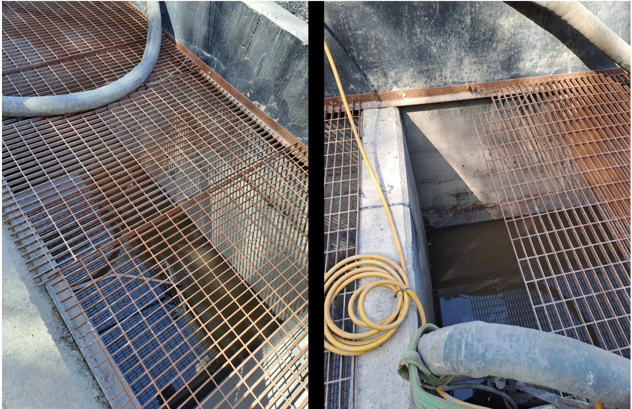
Figure 2 – The site entrance catch pit as observed during the visit.
