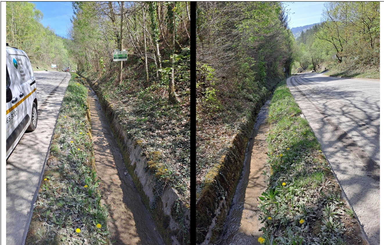
Figure 4 – Site discharge channel as observed during the visit.
