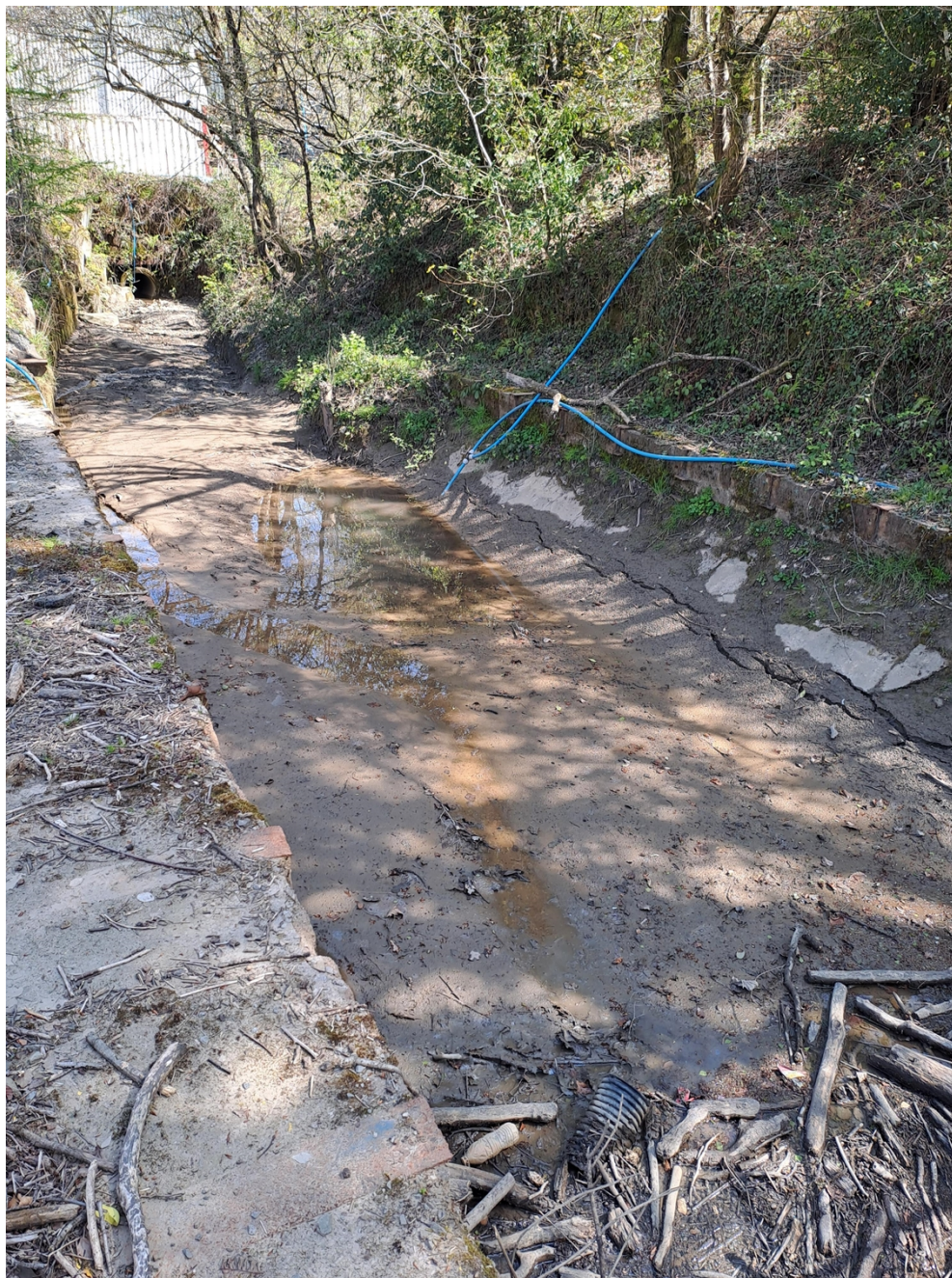
Figure 1 – Final settlement tank as observed during the visit.
