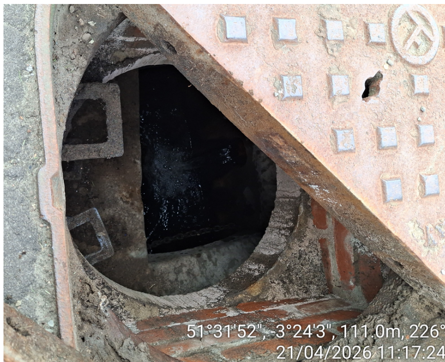
Photo 3: Offsite manhole chamber showing unhindered flow entering surface water
