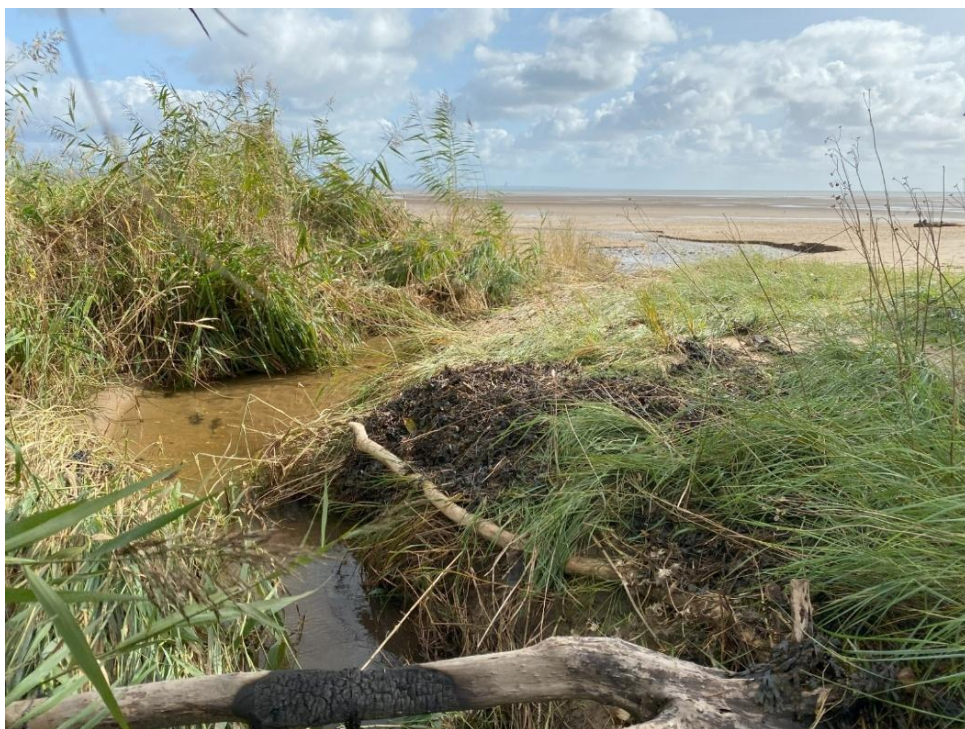
Figure 10-3 - Outfall location - looking seaward showing the channel to be widened
