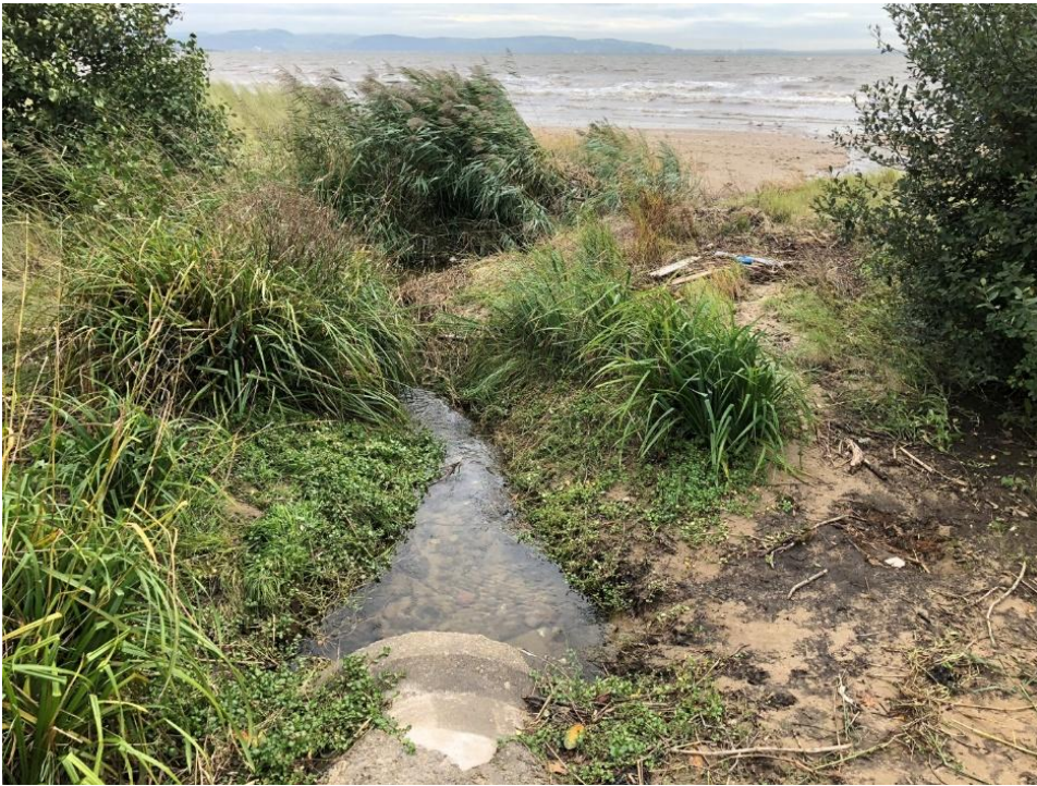
Figure 10-1 - Outfall location - looking seaward showing existing channel
