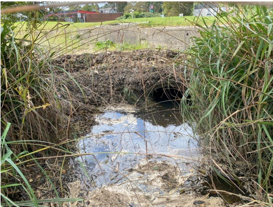
Figure 10-2 - Outfall location - looking inland showing vegetation to be cleared
