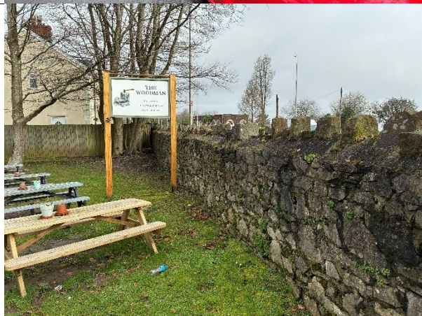
Photograph 5: Stone wall and wooden fence around the boundary of the pub garden area.
