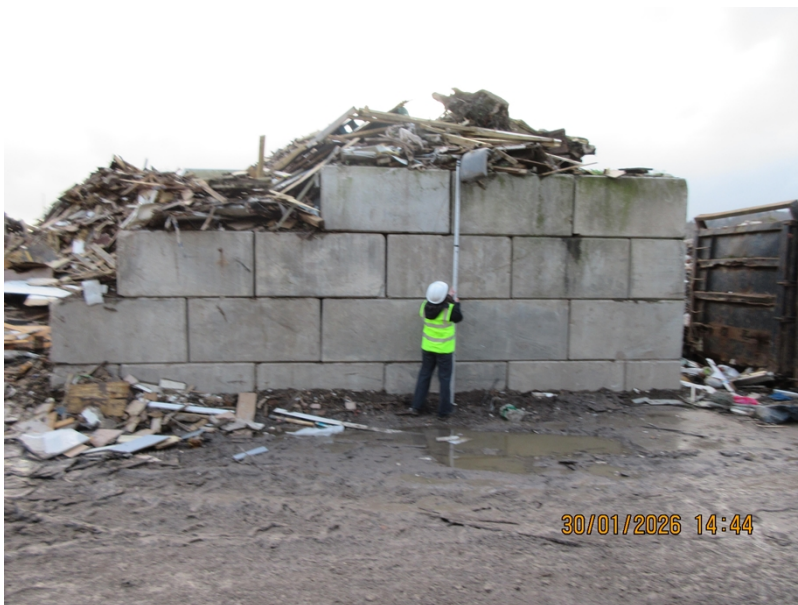
Photograph 3- Wood waste stockpile exceeding the maximum permitted height of 3 meters.
