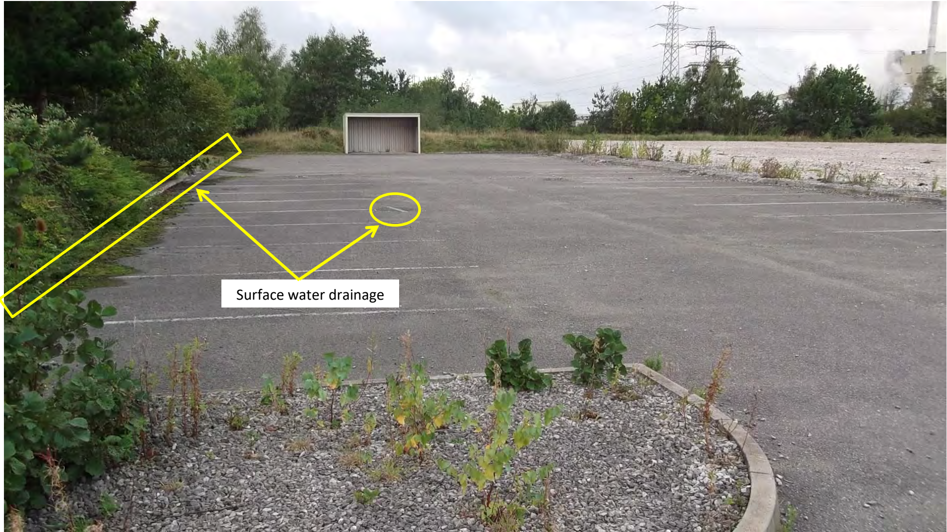
Photograph 3 - Looking westwards on to car park area with surface water drainage. Lateral gully drain present along the southern edge of car park.
