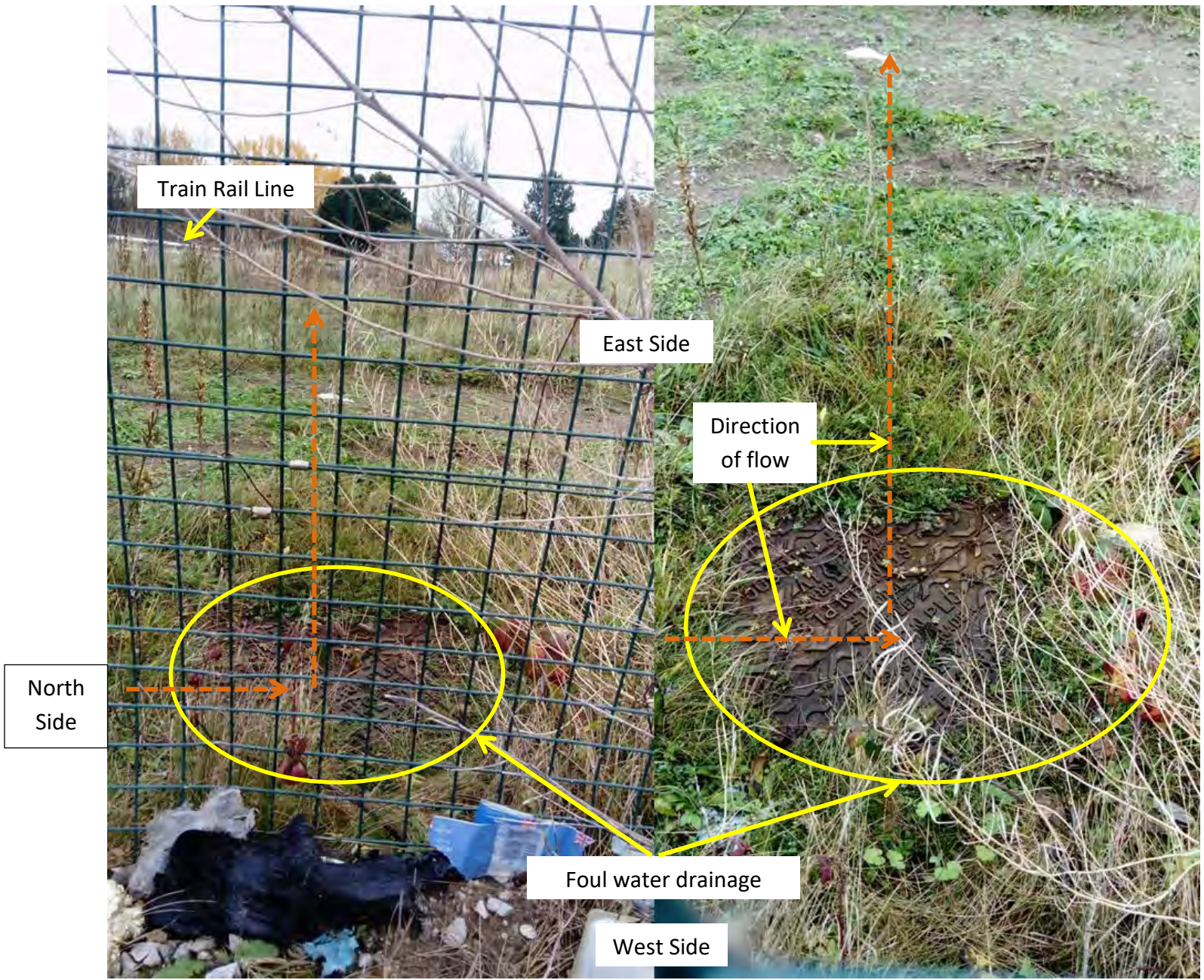
Photograph 15 – Foul water drainage located along the middle of the eastern boundary of the site, draining in a eastward direction towards the train rail line in the background.
