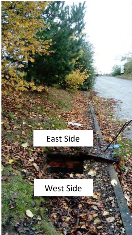
Photograph 5 – Surface water drainage in adjacent to site access ramp. Manhole receiving surface water from the east and proceeding westwards towards the site entrance.
