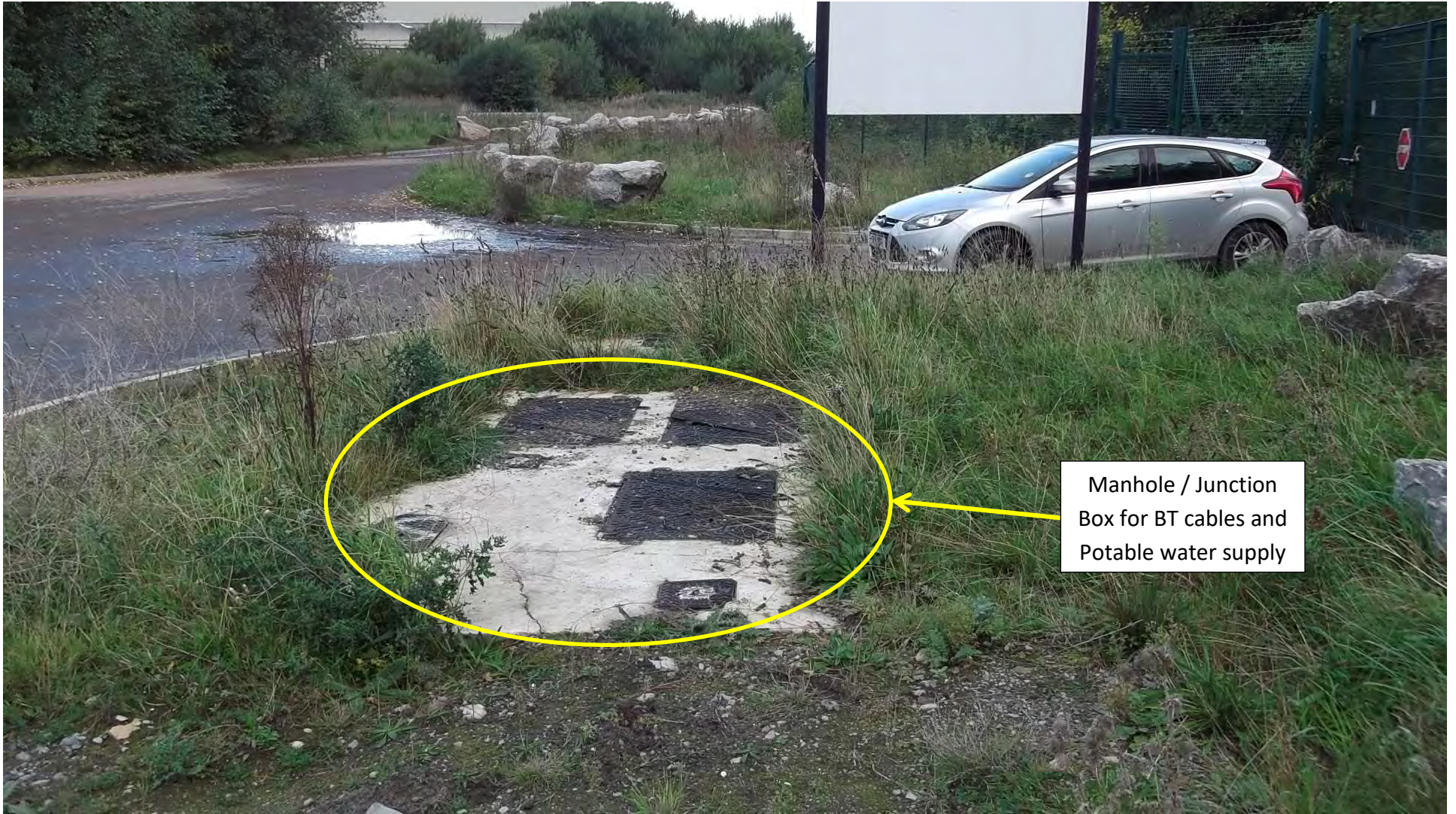
Photograph 29 – Looking northwards at site main access along Weighbridge Rd. Potable water supply and BT cables located along the eastern edge of Weighbridge Rd.
