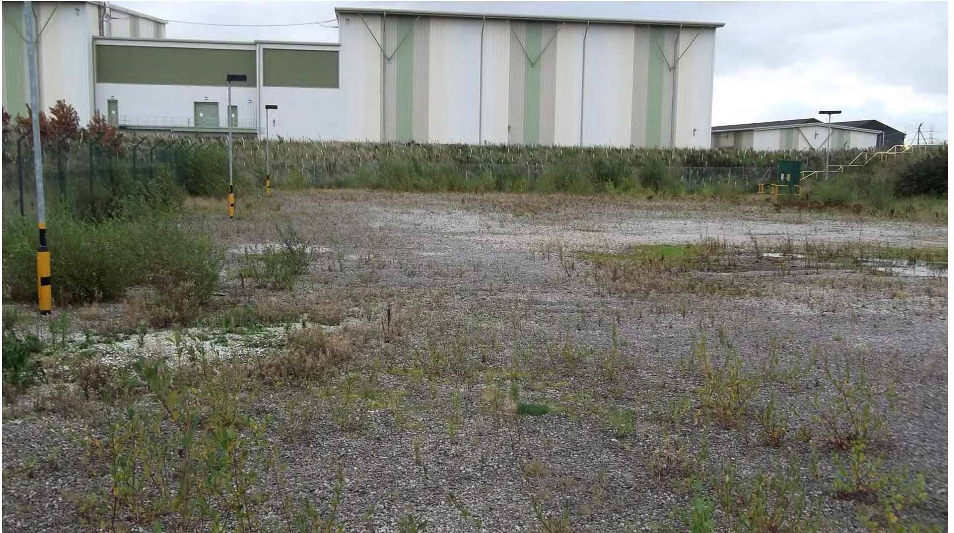
Photograph 24 – Looking southwards on to the Flintshire Bridge Site 400kV Converter Station at the southern boundary of the site. Approximate 3m high earth bund flanking the southern boundary of the site.
