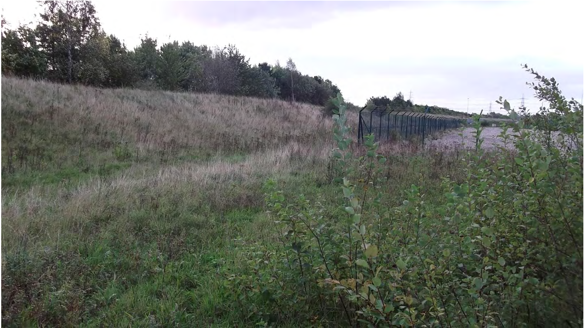
Photograph 20 – Looking southwards along the eastern boundary of site. Approximate 3m high earth bund flanking the eastern boundary of the site.
