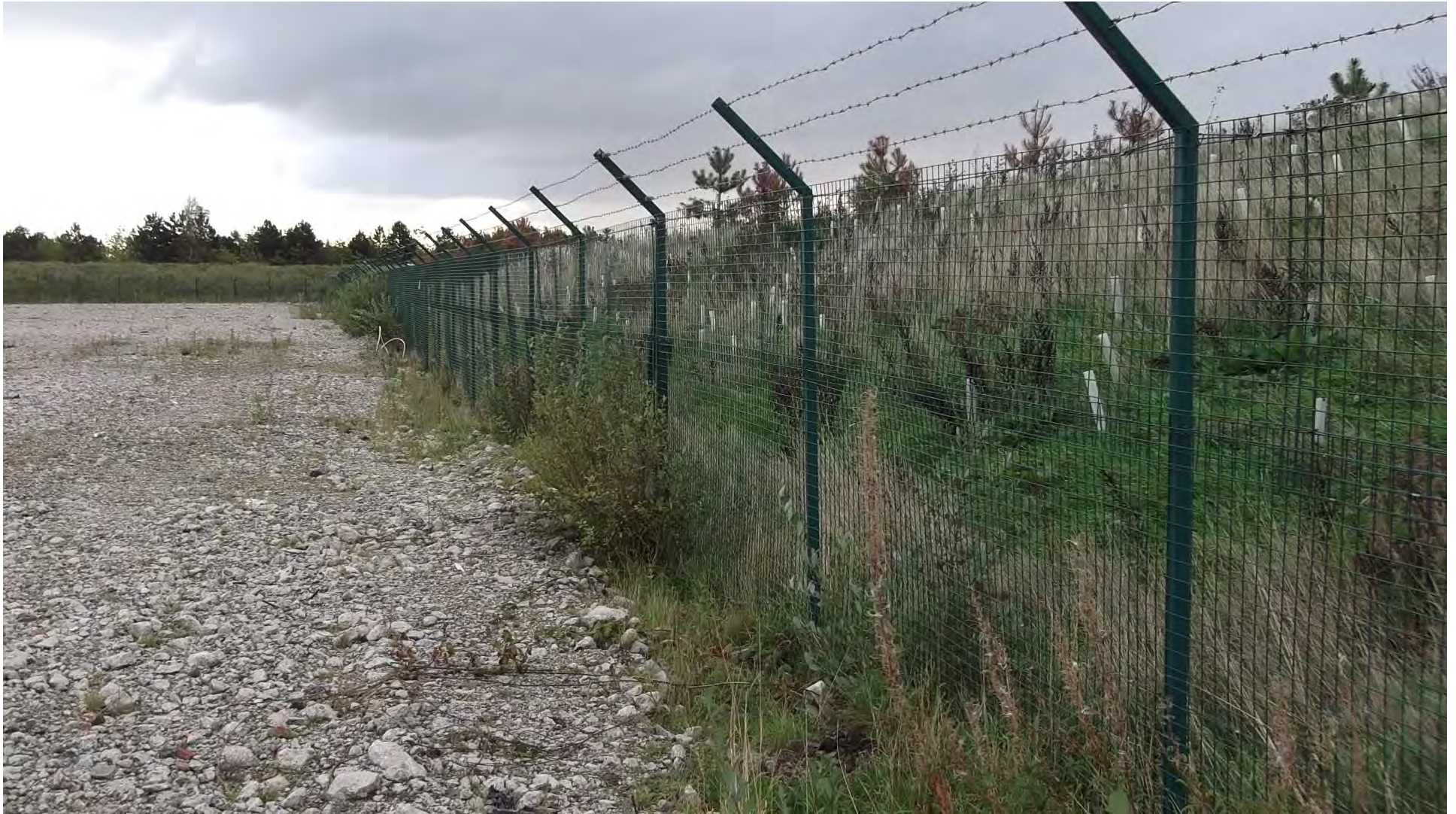
Photograph 23 – Looking eastwards along the southern boundary of the site. Approximate 3m high earth bund flanking the southern boundary of the site.
